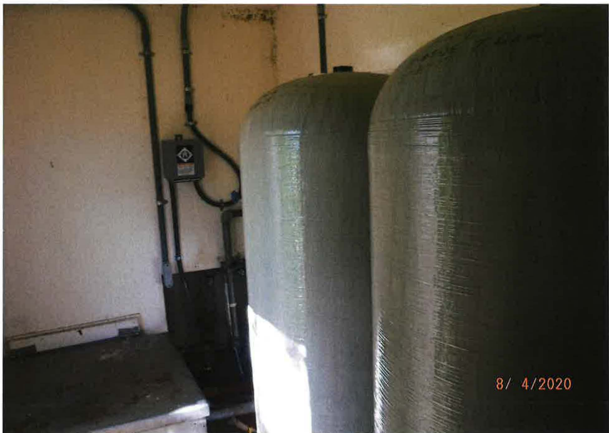
3EA 120 GAL PRESSURE TANKS & 3,000 GAL VAULTED STORAGE CISTERN
