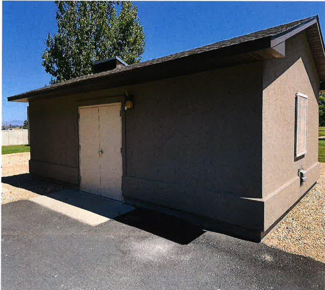
Fig. 2 – 18" well D00030889 w/ 30 hp & 125 hp pumps are located within pump house. Access was not possible during the field exam.
