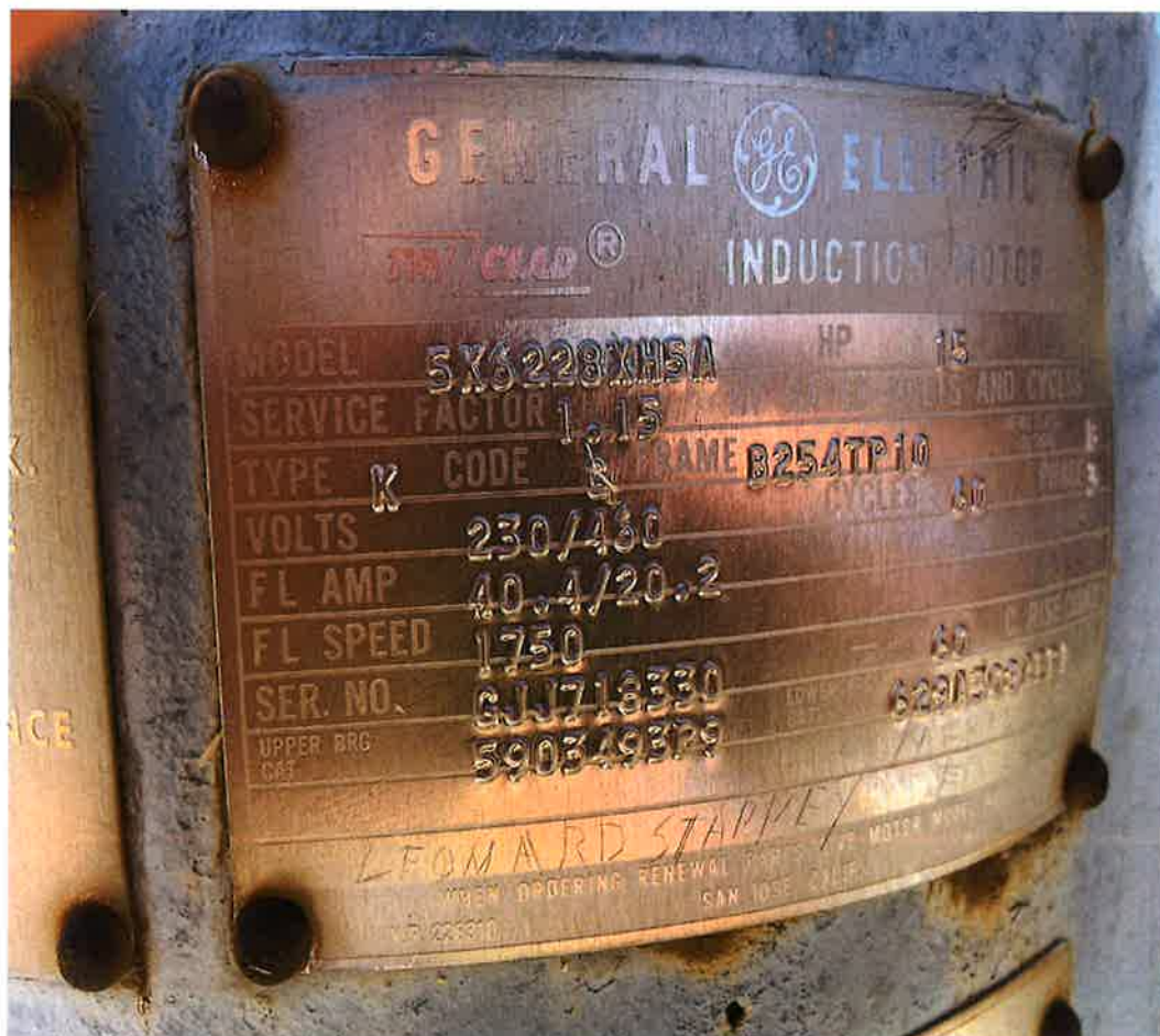
Fig. 6 – Motor info for booster pump:
