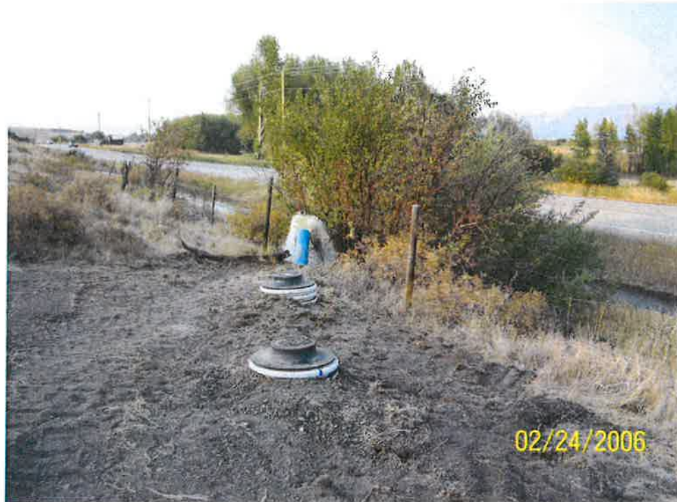
Terminus of the Sam's Hollow mitigation pipeline.
