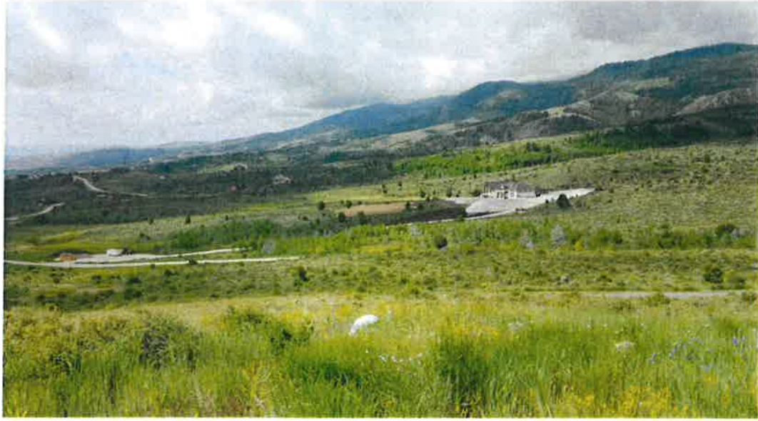
Development that has occurred at Sam's Hollow Water Company as of 2018
