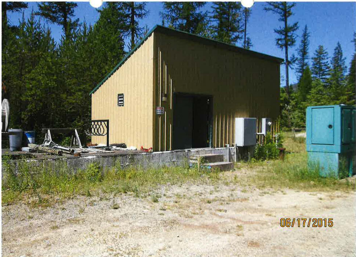
PUMP HOUSE CO-LOCATED WITH 2EA WELLS
