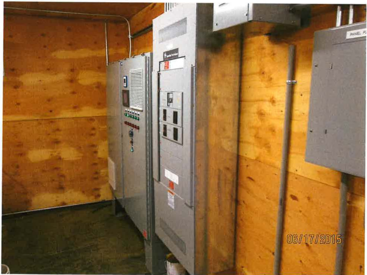
PUMP CONTROL PANEL
