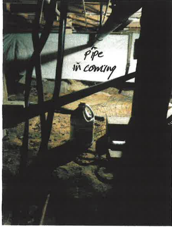
PIPE INTO CABIN
