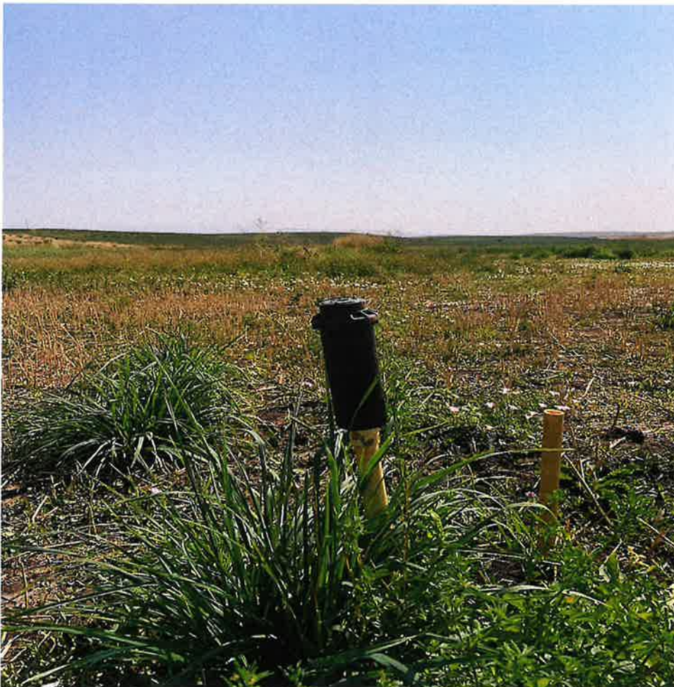
Fig. 6 – Hunter PGP sprinkler heads are used to irrigate NW section of place of use. View looking east.
