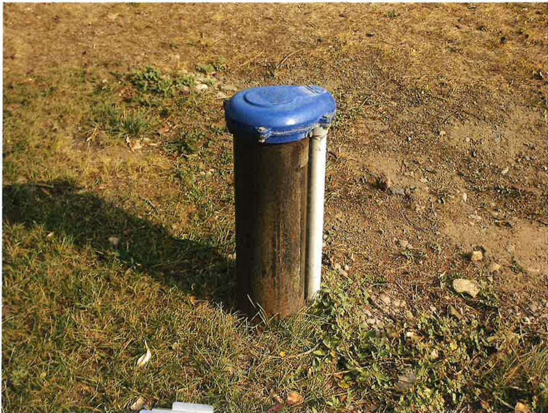
Point of Diversion - well
