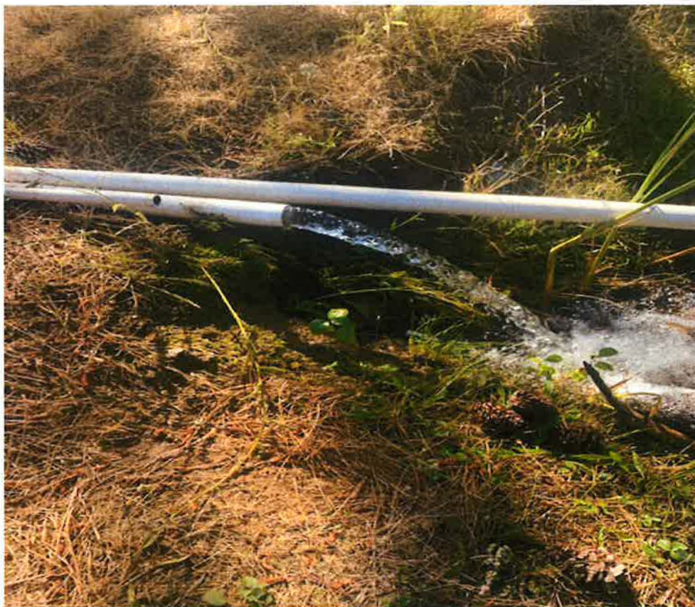
8 HP PUMP DISCHARGING TO 24 HR CONTAINMENT POND
