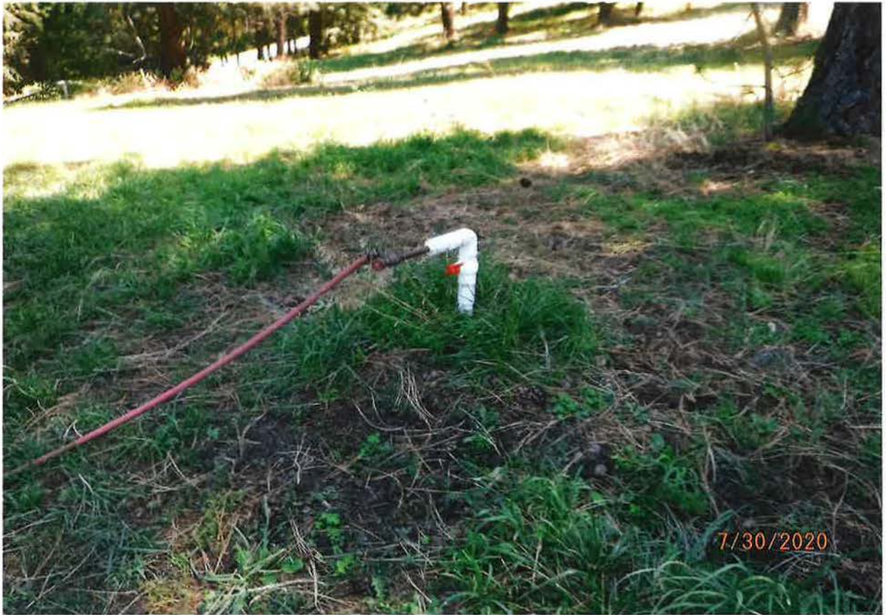
IRRIGATION POU RISER PIPES
