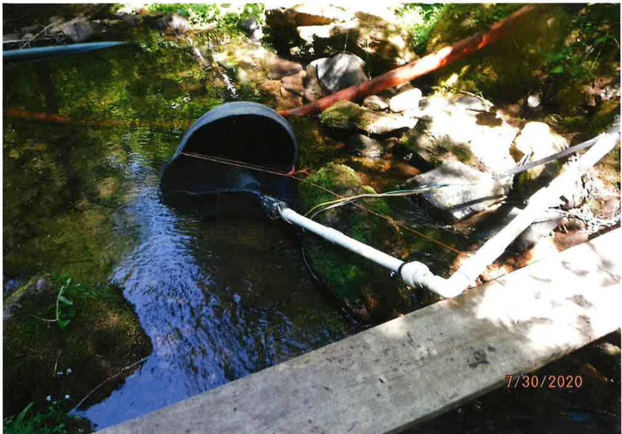
2 ND POD – 2 HP ELECTRIC SUBMERSIBLE PUMP IN CREEK
