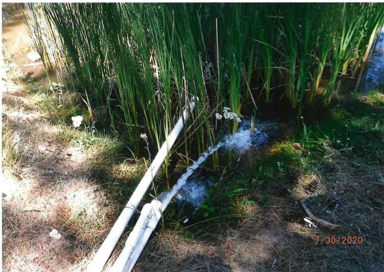
1.5 HP PUMP DISCHARGING TO 24 HR CONTAINMENT POND
