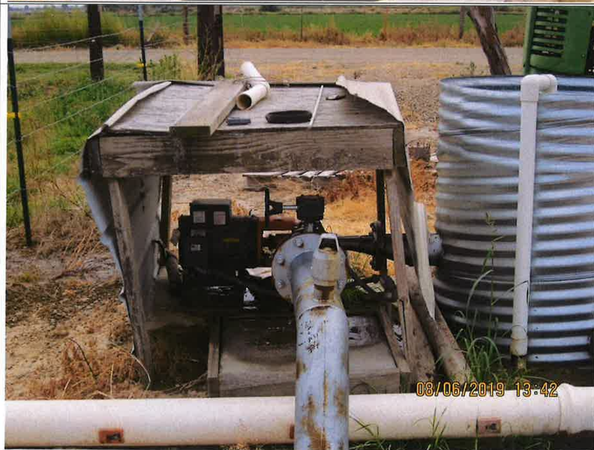
Figure 4. Booster pump attached to holding and pumping out to mainline.
