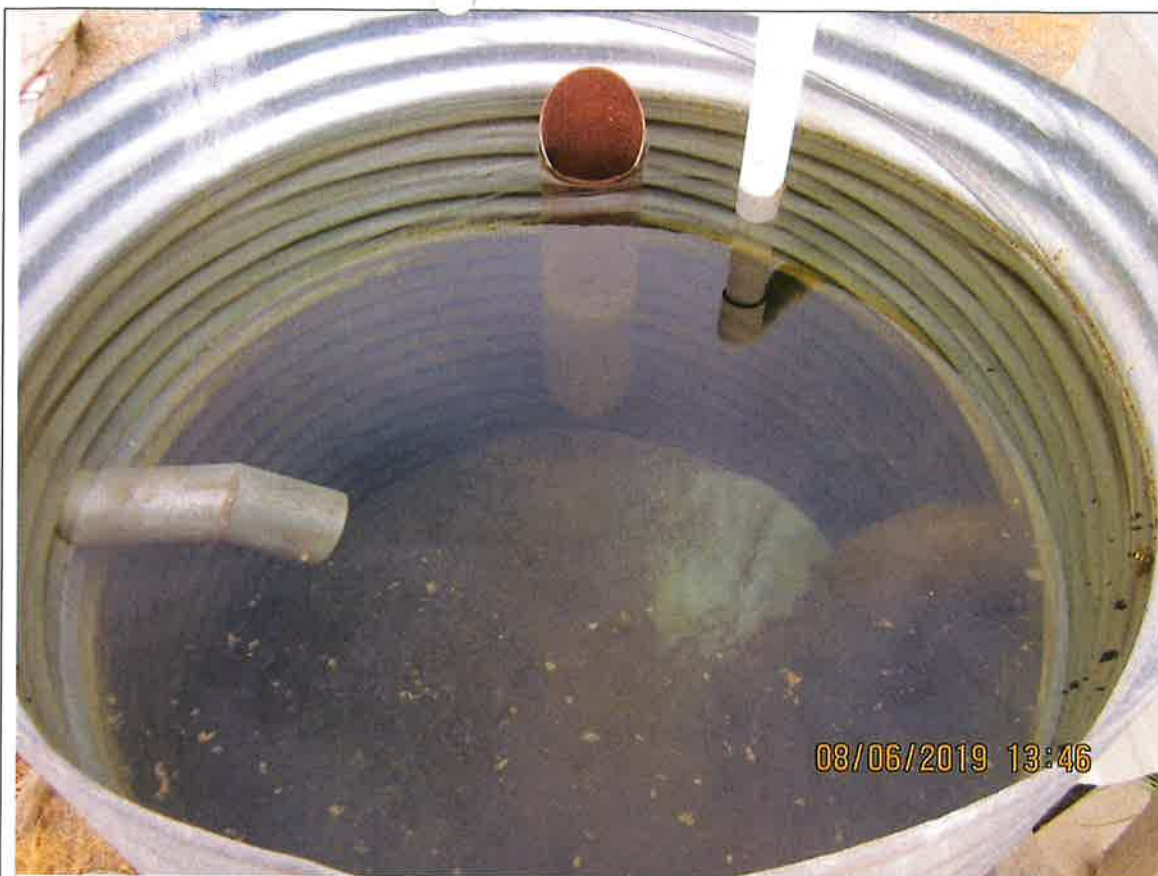
Figure 3. CMP holding tank with overflow pipe, inflow pipe, and outflow to booster pump.
