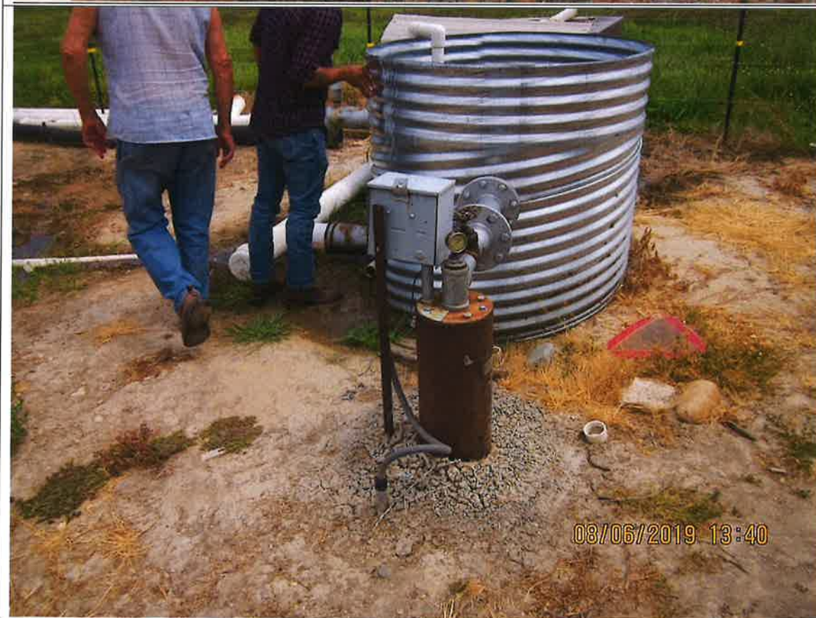
Figure 2. Well pumping into small CMP holding tank.
