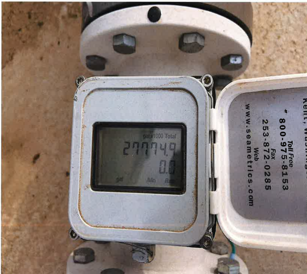
Fig. 8 – The drip station has a Seametrics flow meter installed. Permit holder stated POU is always irrigated at 180 gpm from drip station for crop optimization.
