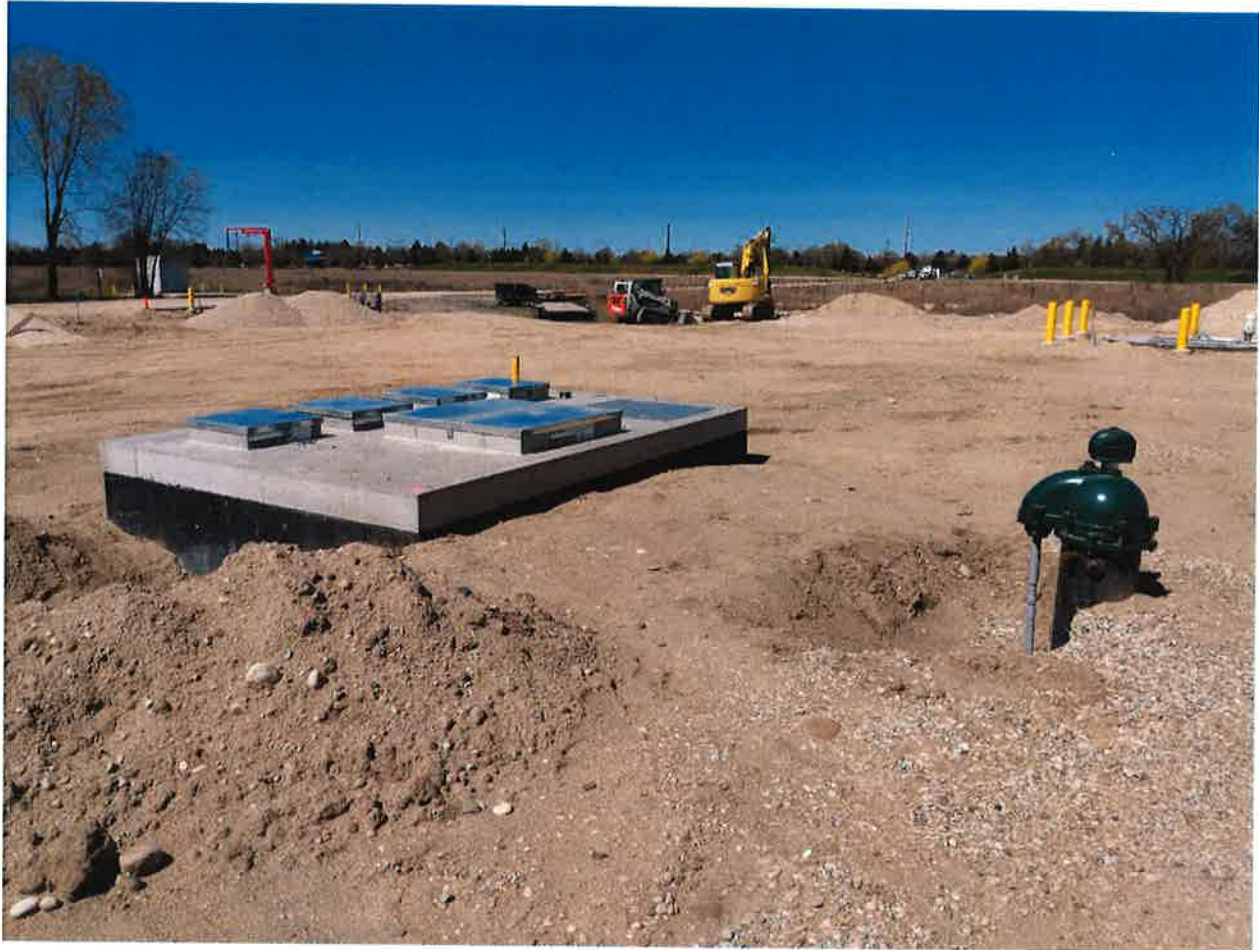
Well head and well piping/valve vault
