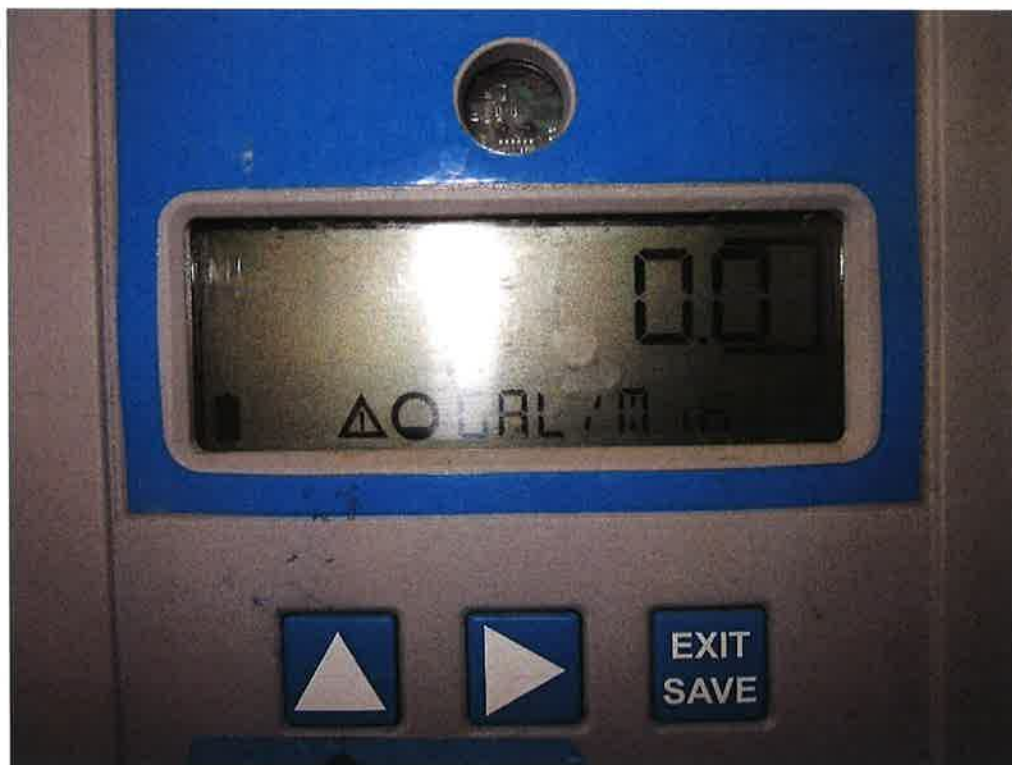
Figure 6: Zero flow on meter at north well, which was the same on south well
