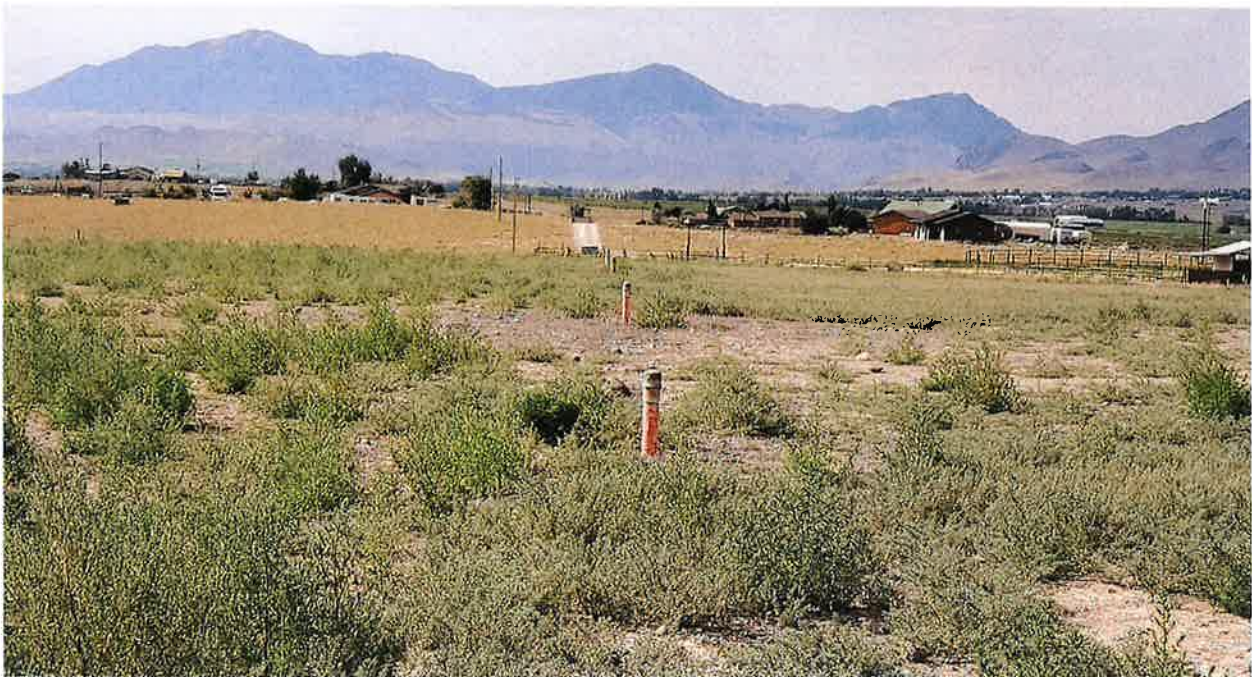
Below: Main line and risers used to irrigate from the hot water well
