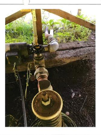
Pump and motor set-up at POD showing 3" suction line heading towards Middle Fork Payette River.
