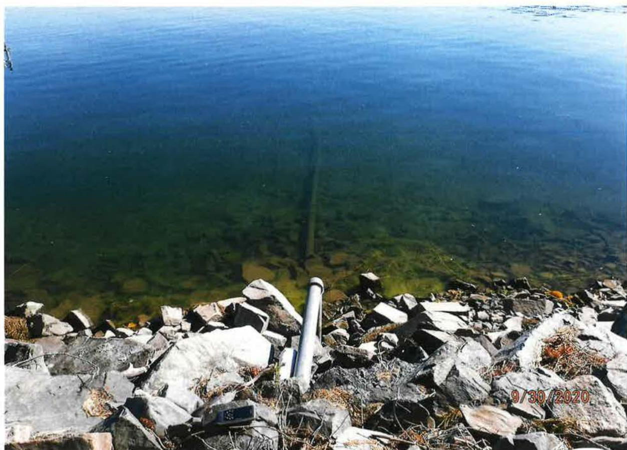
POD -- SCREENED INTAKE PIPE IN THE PEND OREILLE RIVER
