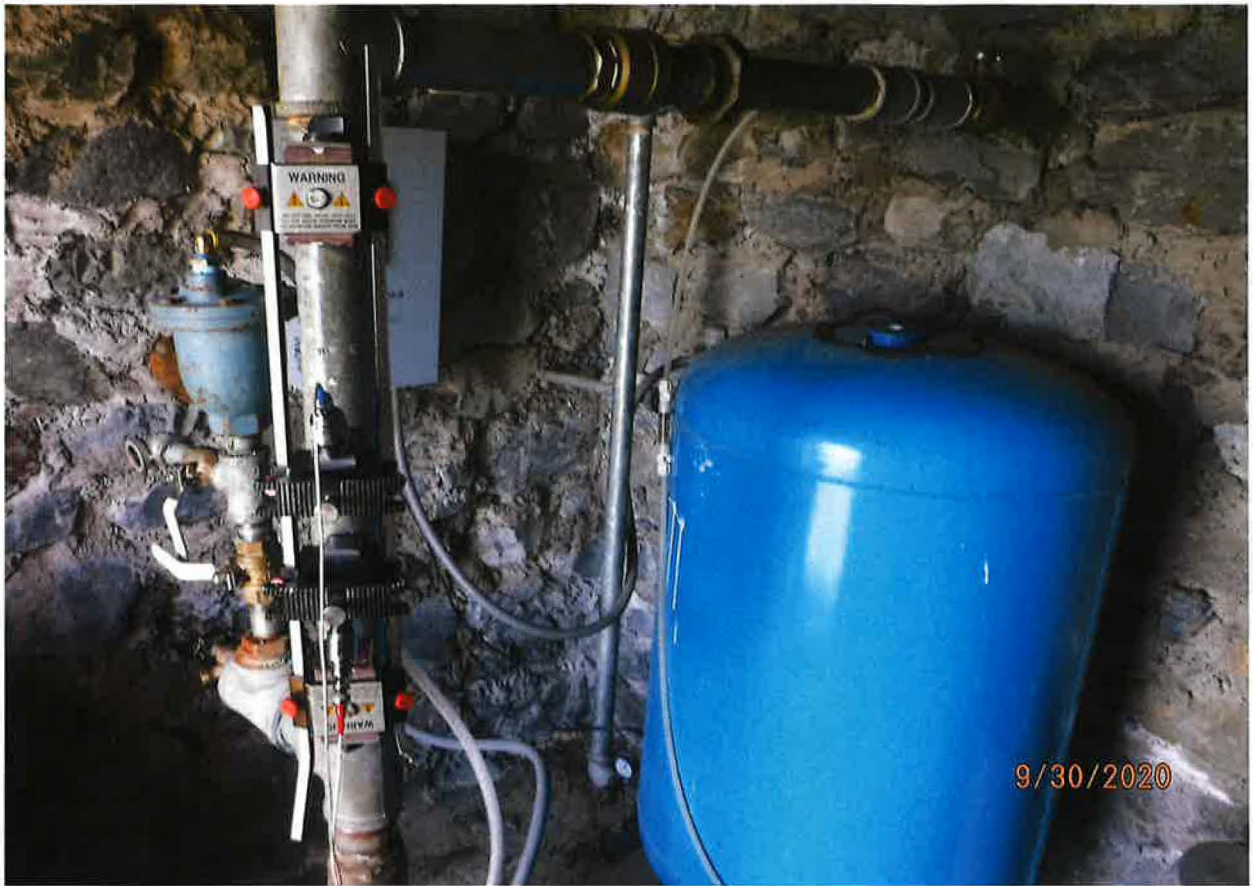
ULTRASONIC FLOW MEASUREMENT TAKEN IN LINE PRIOR TO PRESSURE TANK INPUT TO SYSTEM
