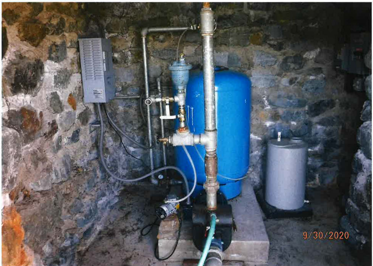
INTERIOR PUMP HOUSE – WATER SYSTEM
