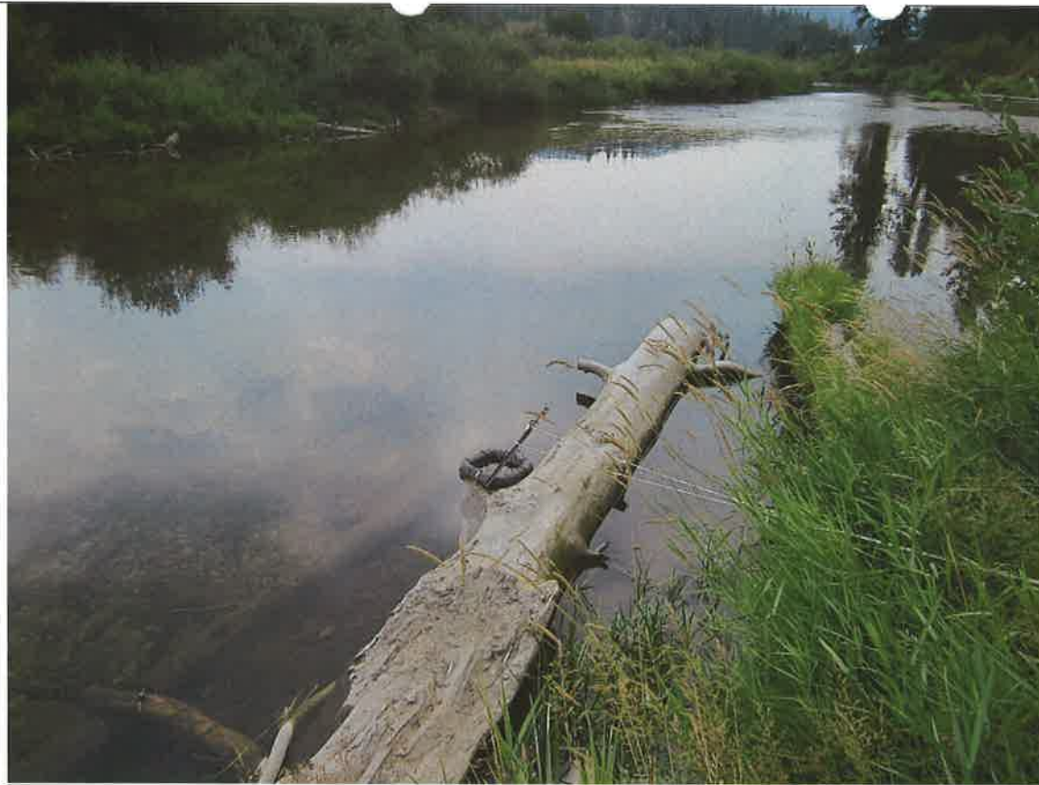
Figure 3. Intake for 2" suction hose.
