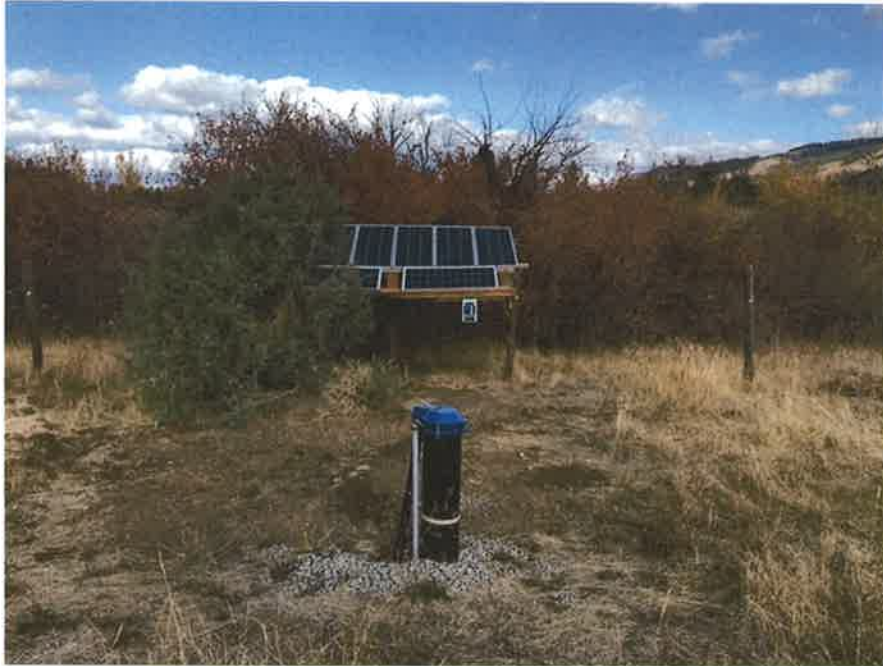
RPS Solar Well Pump, 800 Watt 1.07 hp. Diverts groundwater to aesthetic storage.
