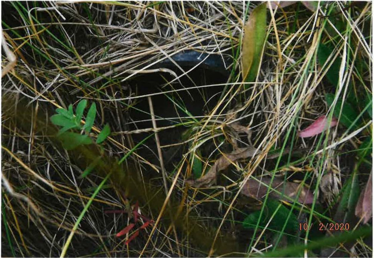
POND OVERFLOW DISCHARGE PIPE OUTFLOW
