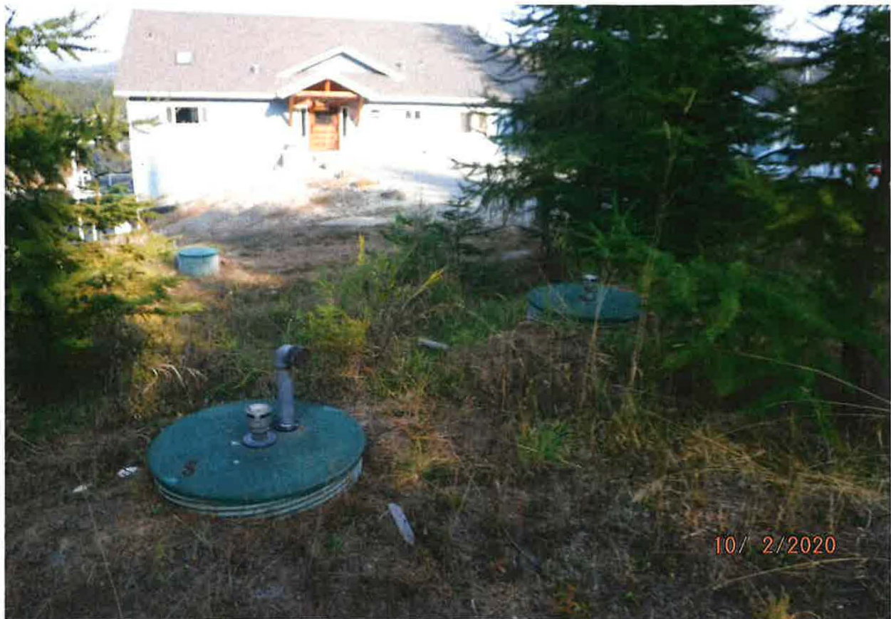
2EA 3,000 GALLON STORAGE TANKS TO SERVICE 2 HOMES OFF WELL
