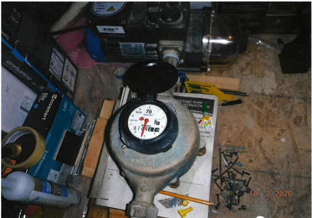
FLOW METER INSTALLED BETWEEN RESERVOIR AND PRESSURE TANK
