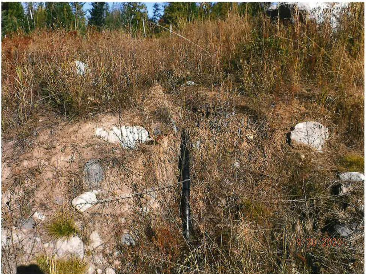
POLY PIPE WATER CONVEYANCE FROM SMALL STORAGE CISTERN TO IRRIGATION FROM STORAGE POU
