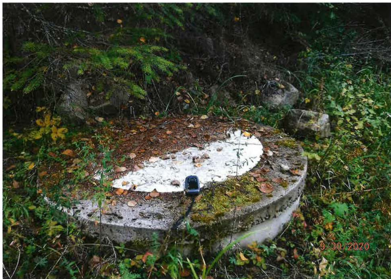
SPRING POD – CONCRETE CISTERN
