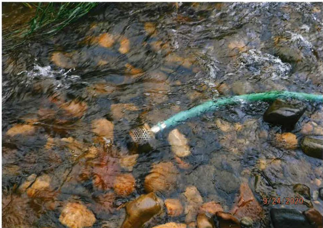
POD – SCREENED INTAKE PIPE IN CREEK
