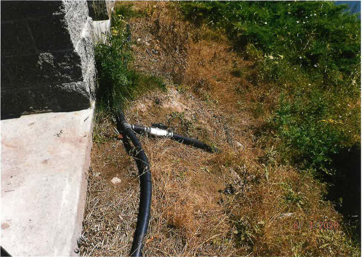
POU – IRRIGATION SYSTEM MAIN POLY PIPE WITH NUMEROUS RISERS FOR ZONES
