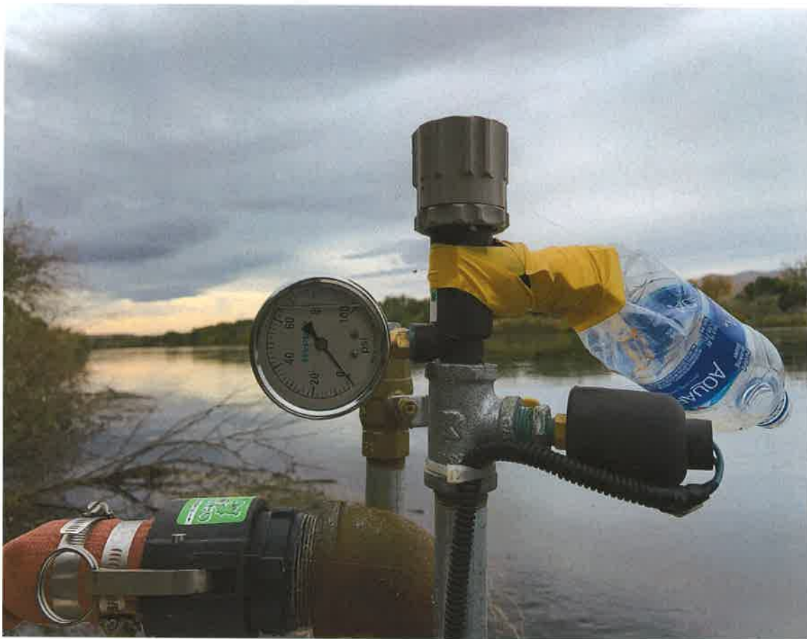
Fig. 5 – Pressure is typically operated at 45-50 psi according to permit holder. Water bottle is for back-pressure.
