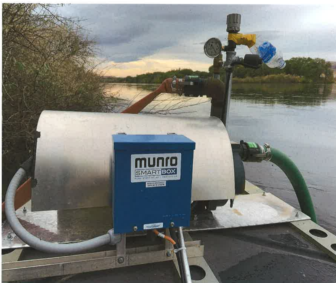
Fig. 2 – Close up view of POD. Pump is covered by metal sheet and controlled via Munro smartbox.
