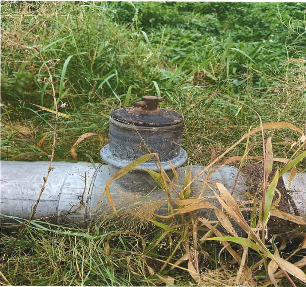
Fig. 7 – 4" PVC connects to 6" mainline. Hand-lines are attached to mainline at these valves.
