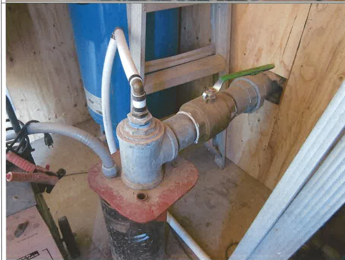
Figure 2. Well head inside pump house.
