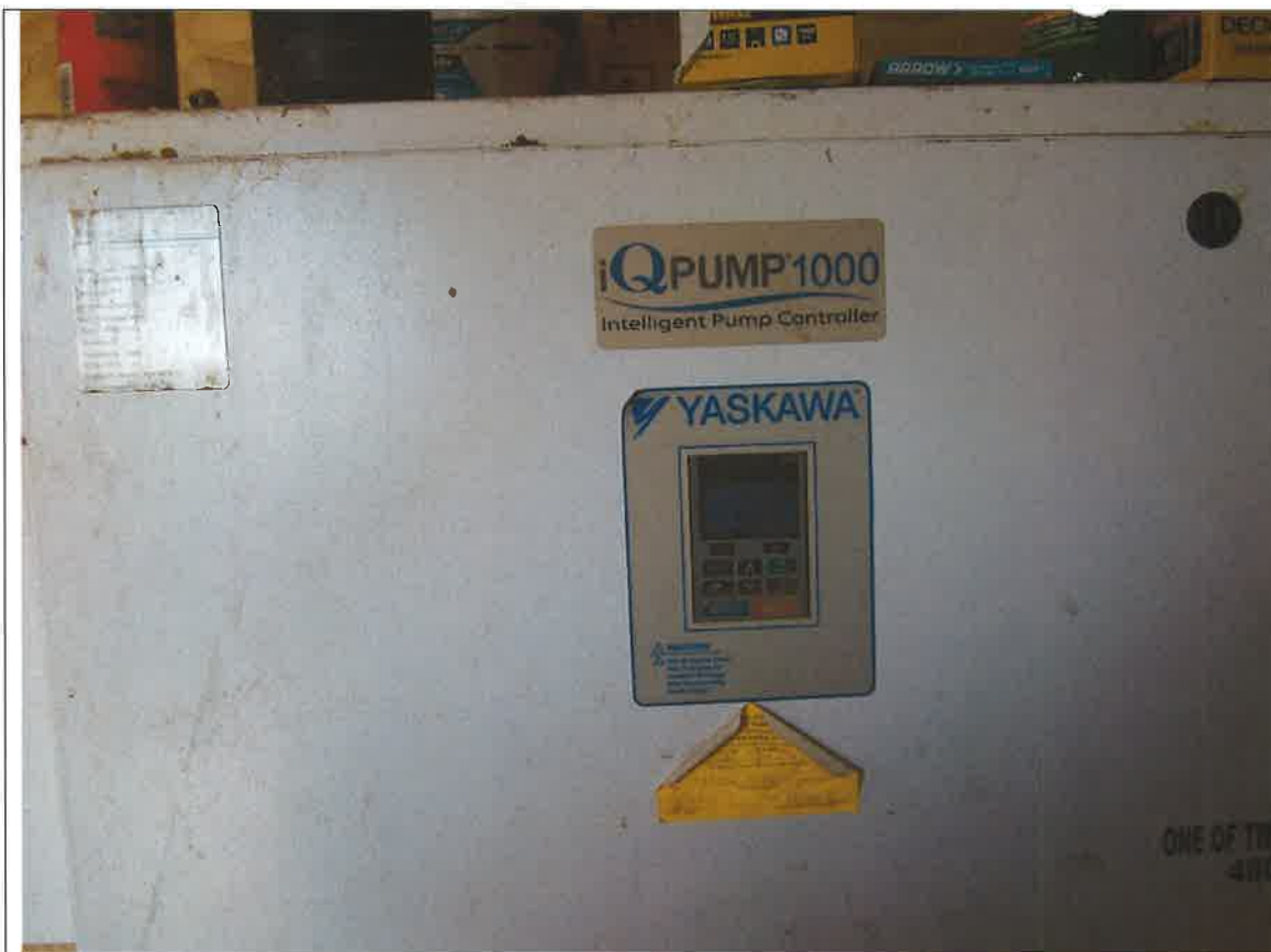
Figure 3. Yaskawa iQPump 1000 pump control panel.
