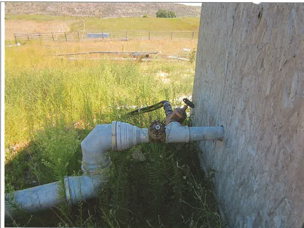
Figure 5. Pipeline exiting pump house and expanded to 8-inch aluminum mainline.
