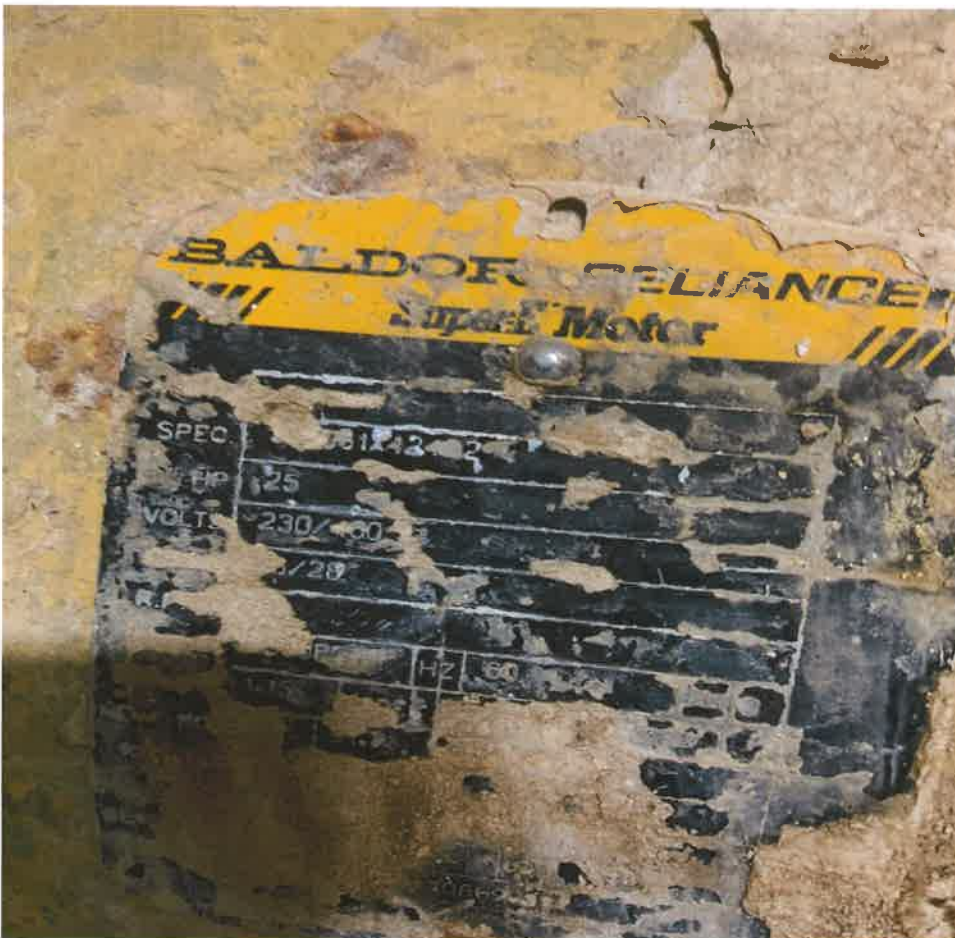
Fig 12 – Motor/pump information for booster pump was corroded. Only discernable information was 25 hp and 230/? Volts.
