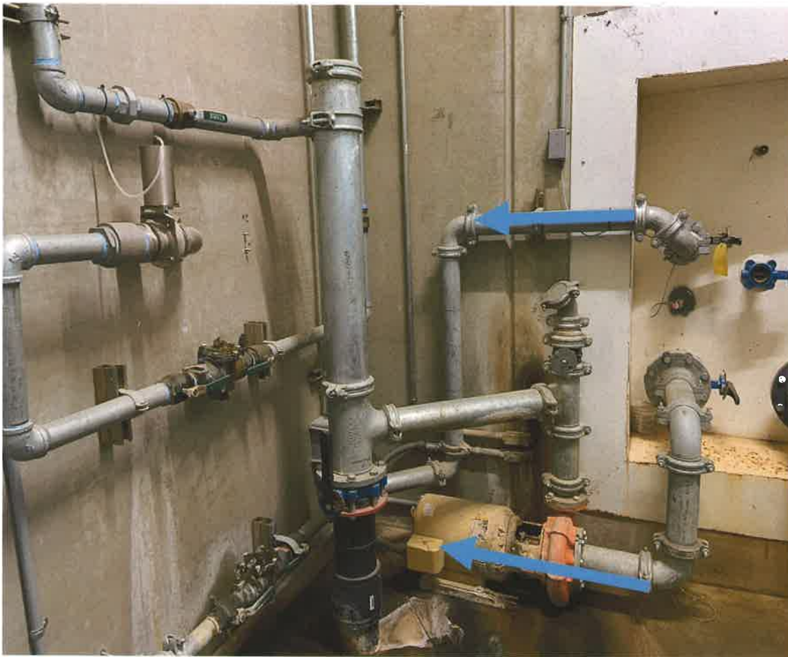
Fig 11 – Booster pump for water leaving holding tank seen in bottom right.
