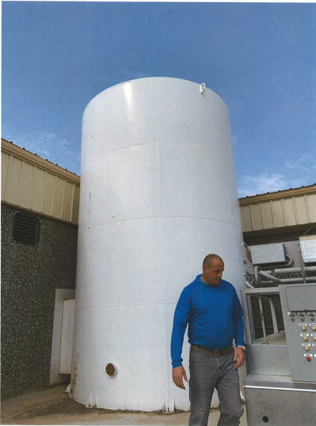
Fig. 13 – Roughly 12,000 gal holding tank, which was about 24' tall. Tank is usually held 1/3 to 2/3 full according to employees.
