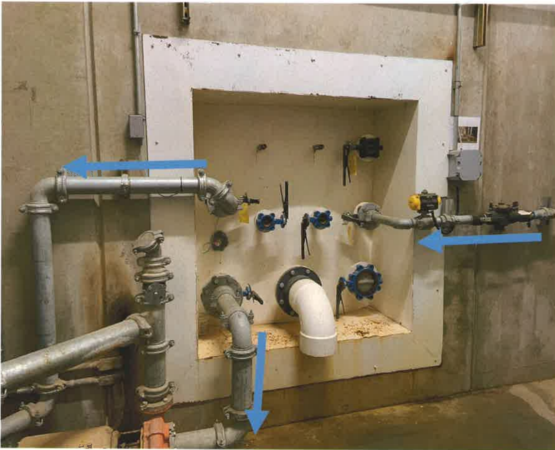
Fig. 9 – Water flows into holding tank from well via pipe on right side of picture, then out via upper left pipe to milking barn and via lower left pipe to corrals.
