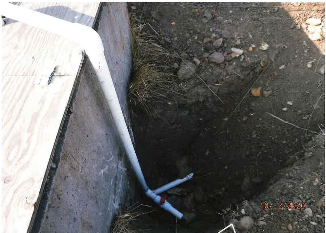
POD – WATER PUMPED FROM CISTERN WHEN IT RECHARGES TO STOCKTANK
