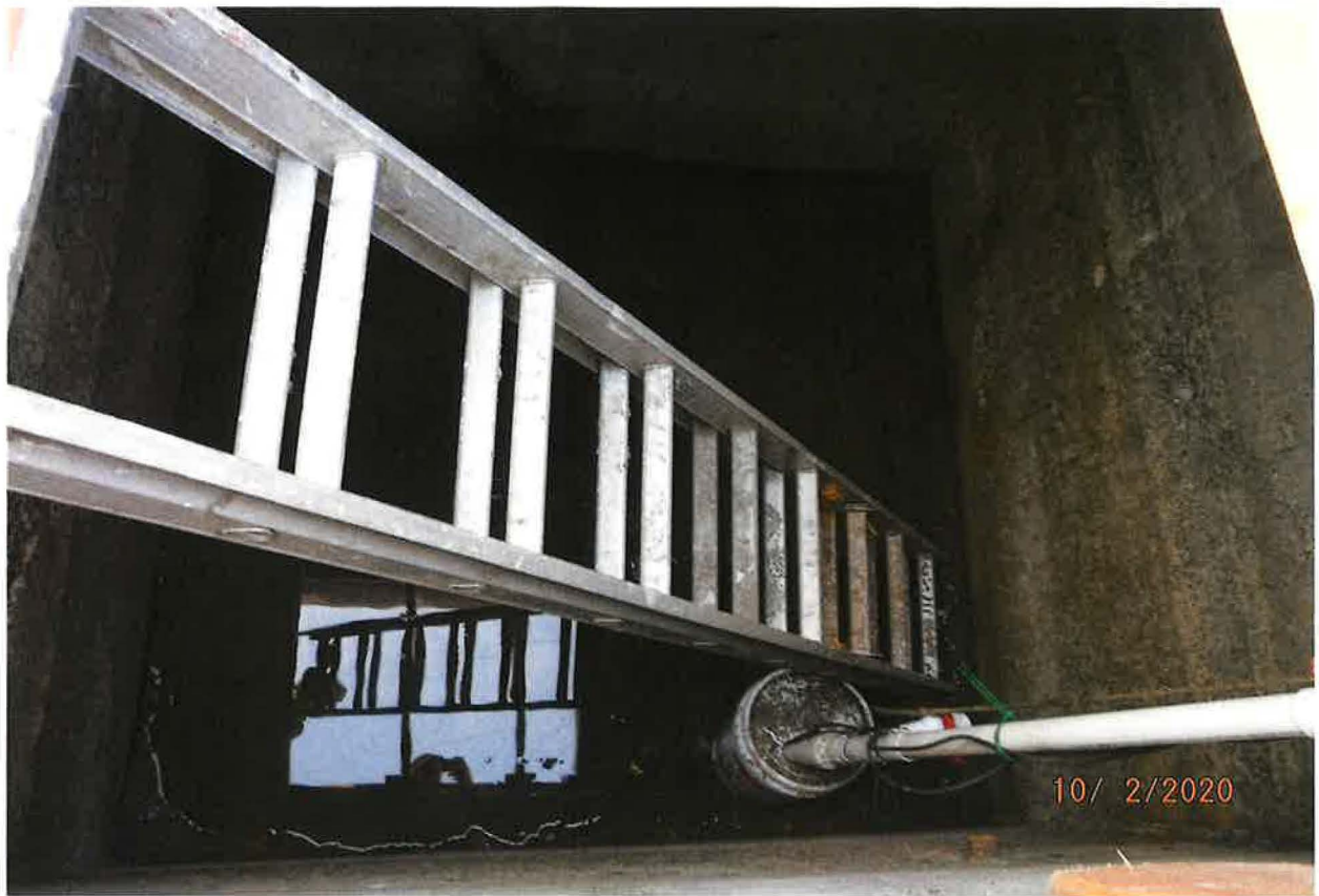
POD – CONCRETE CISTERN 8 FT X 8 FT X 8 FT – FILLS THROUGH CRACKS IN FLOOR
