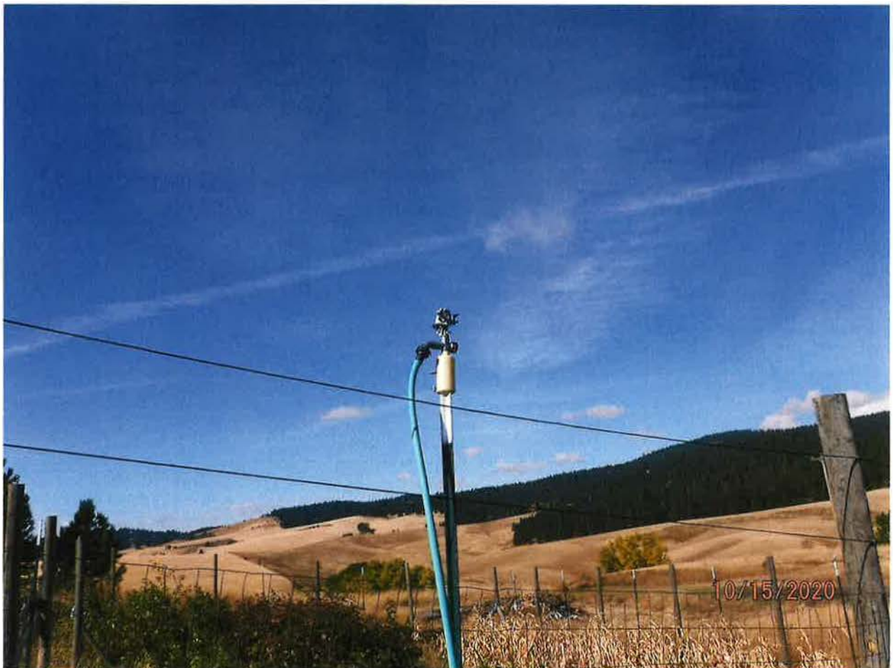
FIRE HOSE FROM POND TO HOSE CONNECTION FOR SPRINKLER IRRIGATION FROM STORAGE USE
