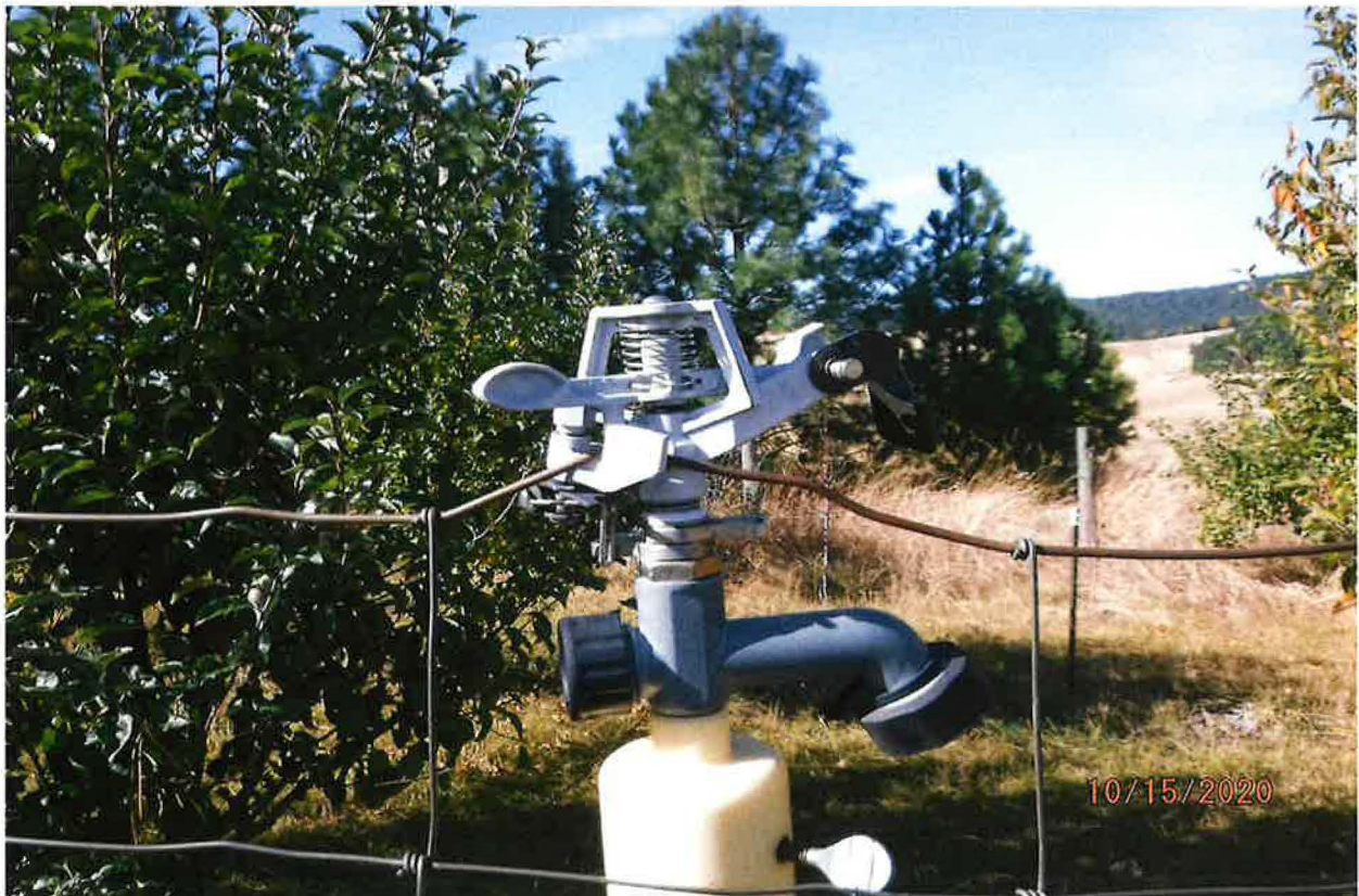
IRRIGATION FROM STORAGE POU – 6 EA SPRINKLERS MOUNTED ON GREEN METAL FENCE POSTS
