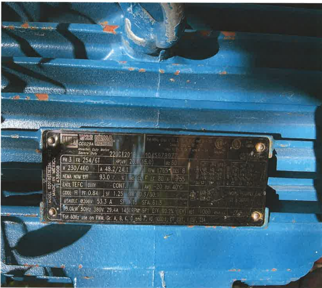
Fig. 4 – Motor info for right pump:
