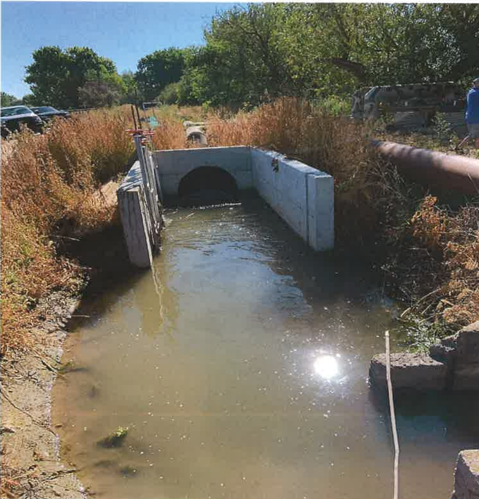
Fig. 12 – View looking east, opposite of Fig. 11. Water flows from pump into ditch, then into subsequent ditches via headgates to left. Overflow water is diverted back to Boise River via pipe in bottom right corner of picture.
