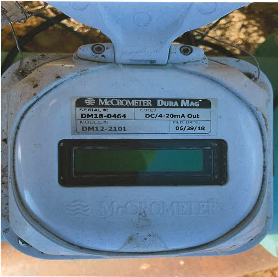
Fig. 9 – An additional McCrometer measuring device was installed off of the right pump for when the diversion output is switched. It was not used during the field exam. McCrometer info:
