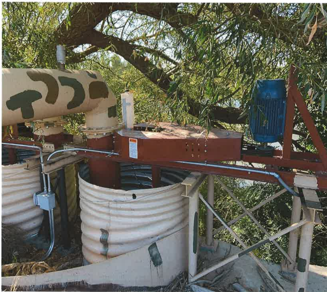
Fig. 2 – Close up view of right diversion pump and pipe. Diversion GPS at: 43° 43' 39" N 116° 51' 16" W
