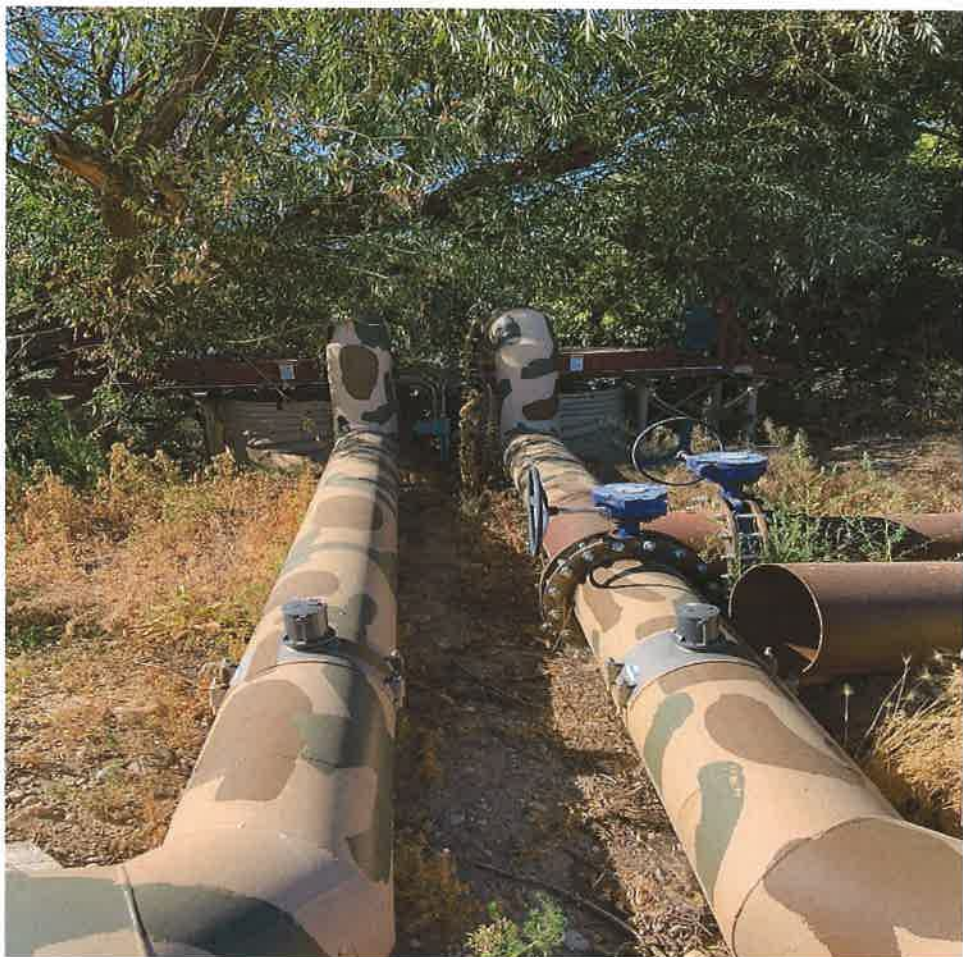
Fig. 1 – Two pumps in background and measuring devices in foreground looking south. Control box is located to the right of picture and is lockable.
