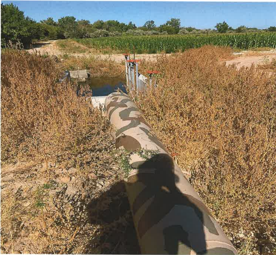
Fig. 11 – View looking west for one of two pipes off of right pump. Water flows north through headgates to ditches via this pipe and straight west under the road via other pipe.
