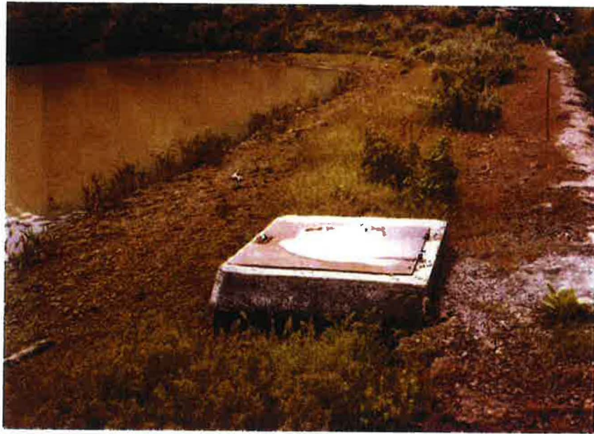
Outlet control box, locked
