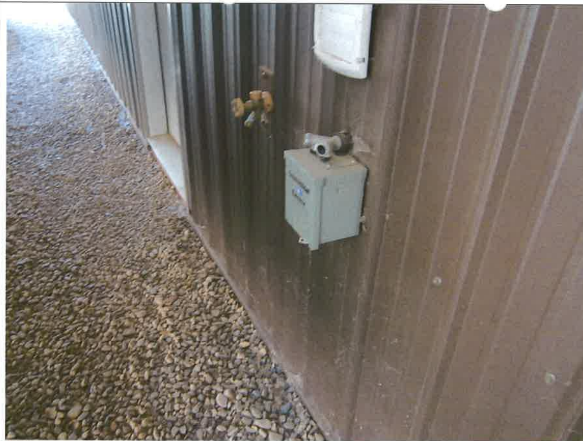
Figure 5. Frost free spigot on shop.
