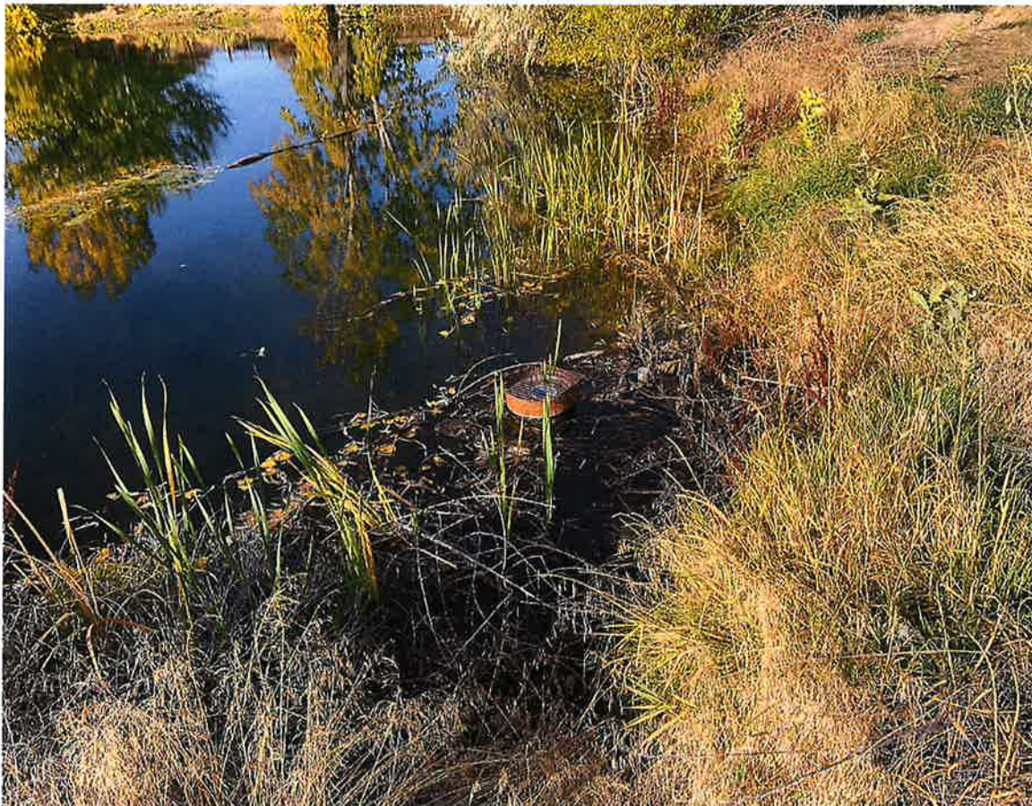
Fig. 6 – Overflow pipe in the NW corner of storage pond flows into retention pond north of this pond.
