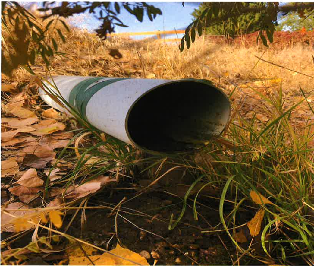
Fig. 3 – Groundwater is pumped into pond via this pipe and then flows down the natural slope into the pond.
