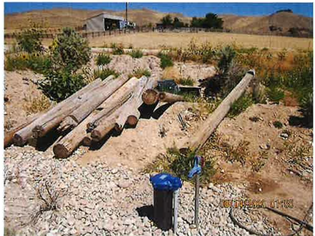
Well head in foreground with storage tank in background.
