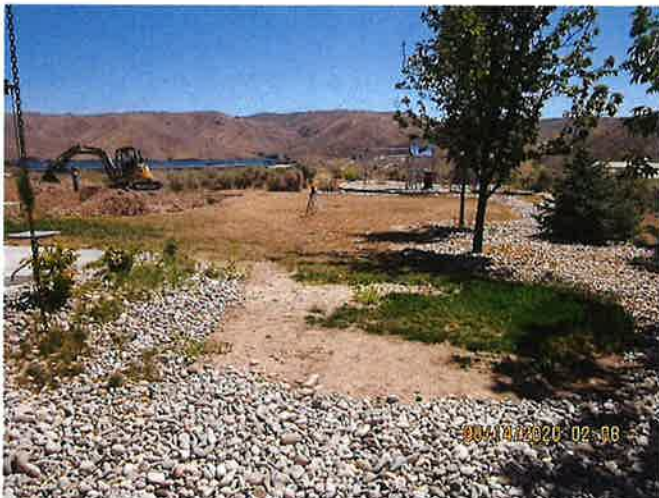
Irrigation occurring on SW side of home. Pool being excavated in background.
