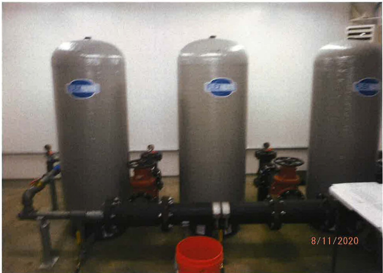
WATER CONVEYANCE SYSTEM
