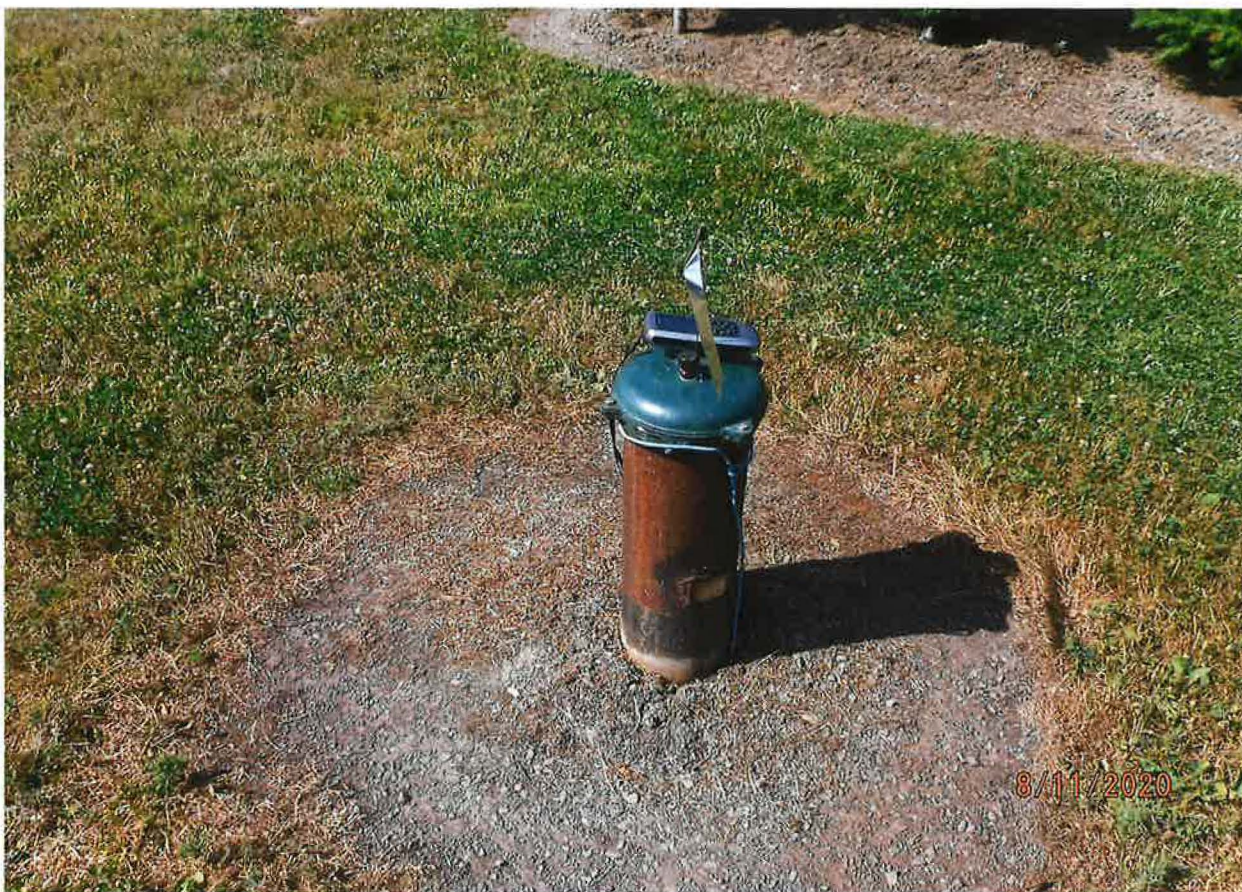
POD – WELL No. 2 D0051750
