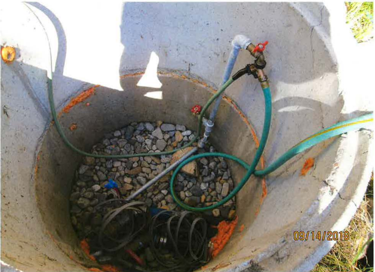
WATER CONVEYANCE SYSTEM – PUMP SYSTEM DRAWING WATER FROM POND
