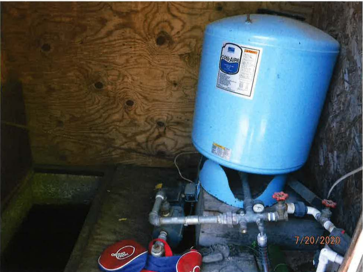
SHED WITH 24HR USE STORAGE CISTERN IN FLOOR AND PUMP HOUSE
