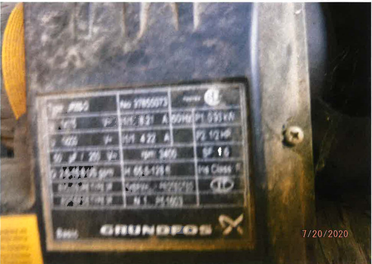
1/2 HP GRUNDFOS PUMP FROM 24HR STORAGE CONTAINMENT TO POU USES
