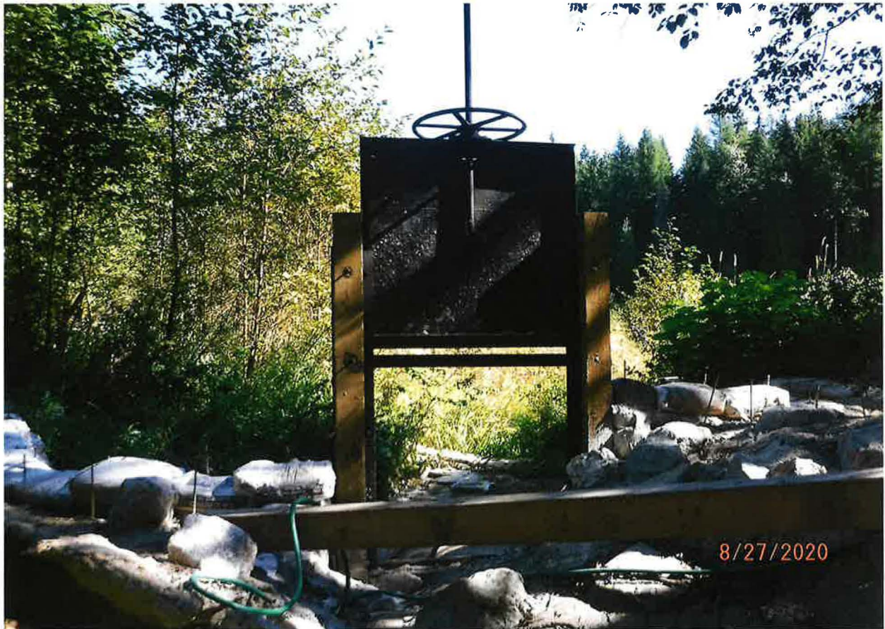
POD - DAM WITH HEADGATE (BEING REPAIRED FROM SPRING BLOW-OUT)
