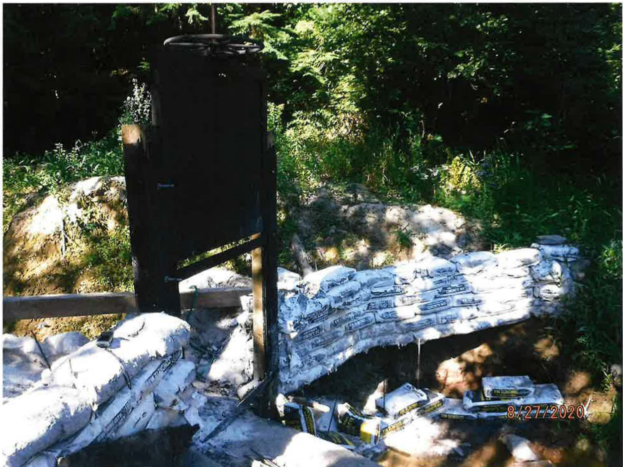
POD - DAM WITH HEADGATE (BEING REPAIRED FROM SPRING BLOW-OUT)
