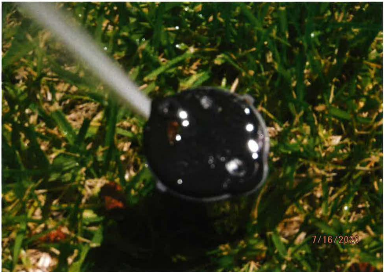
RAINBIRD PRESSURIZED IRRIGATION SYSTEM - 1.5 NOZZLE SIZE = 1.5 GPM PER SPRINKLER
