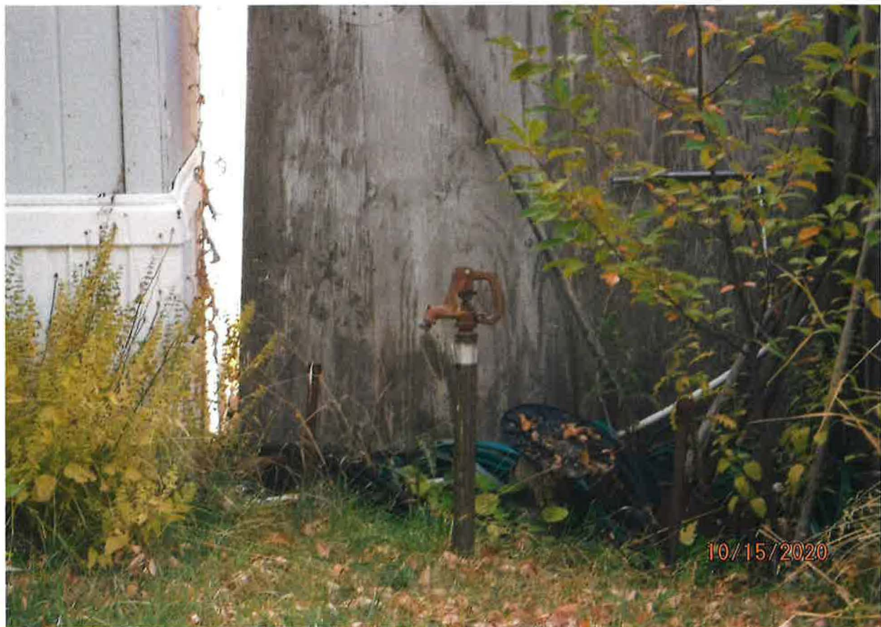
DOMESTIC POU – FROST FREE HYDRANT AT EACH MOBILE HOME SLIP
