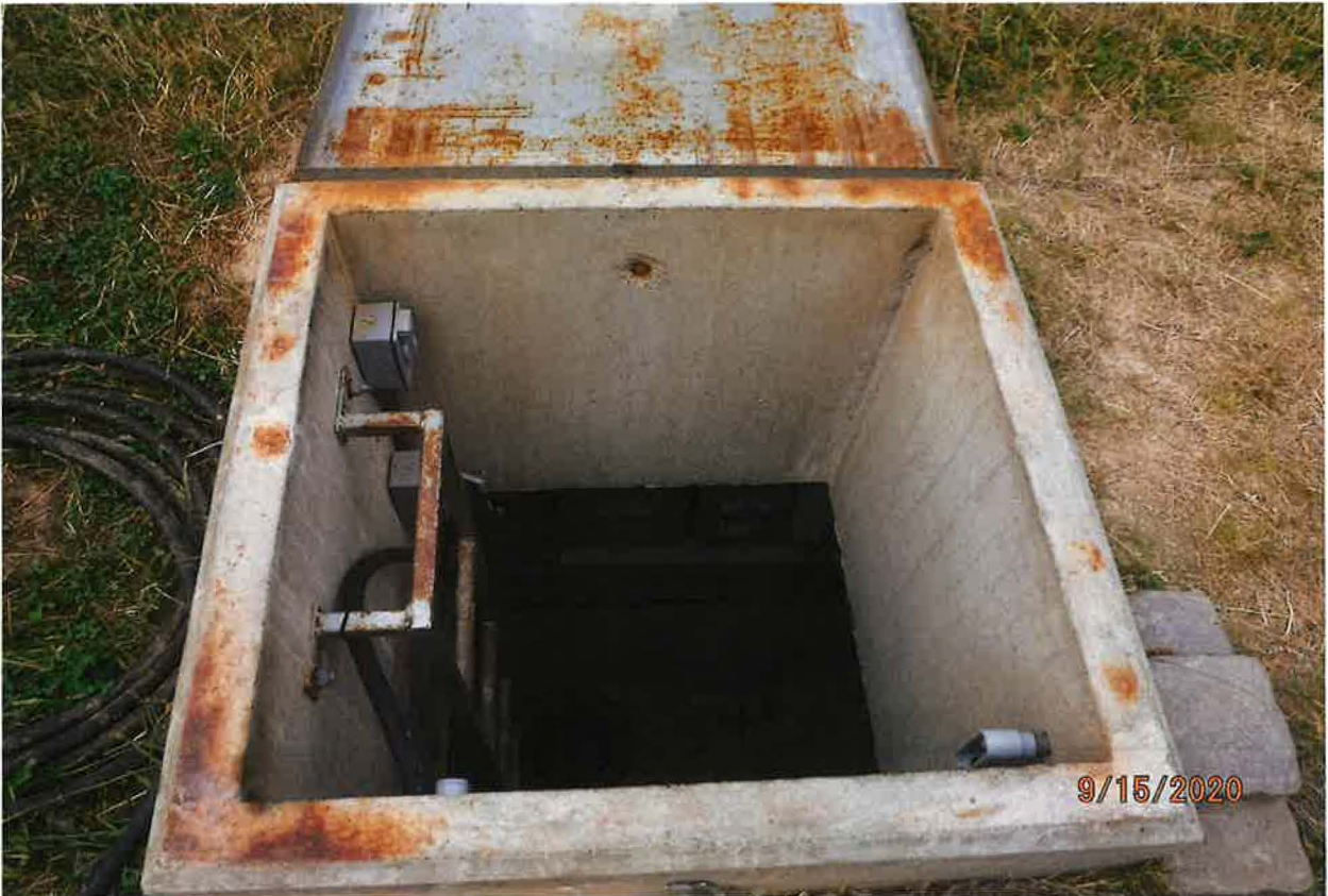
WATER SYSTEM PUMPING CONTROL VAULT
