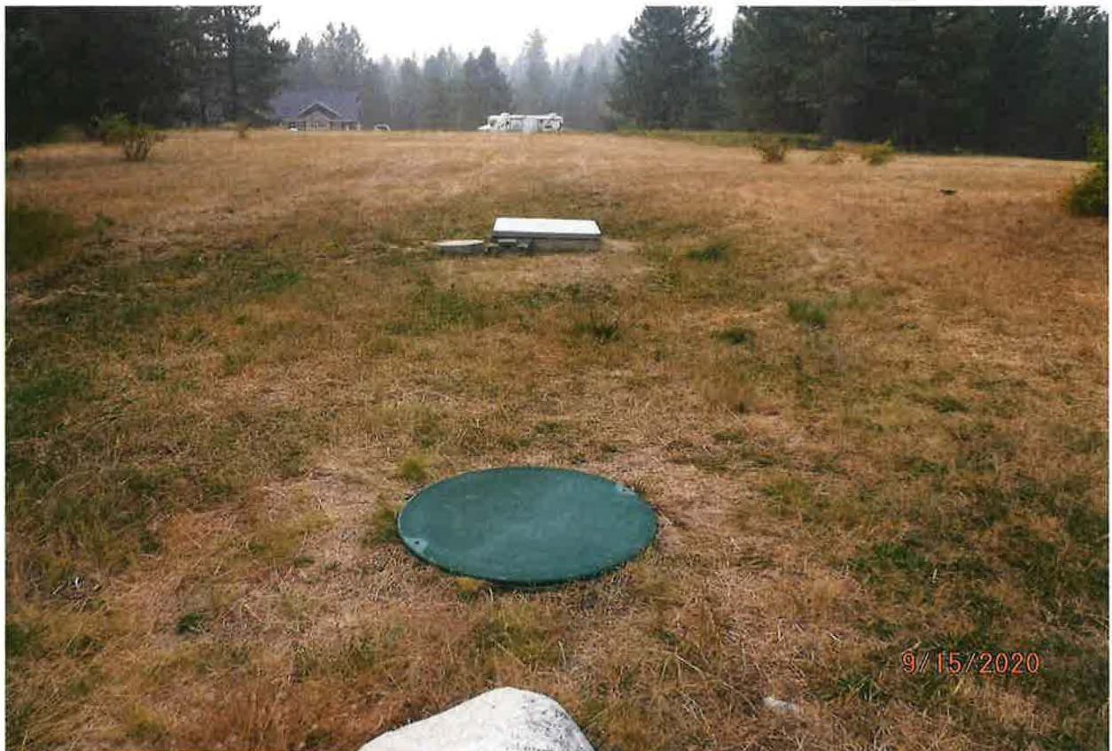
1EA 3,000 GALLON COMMUNITY WATER RESERVOIR
