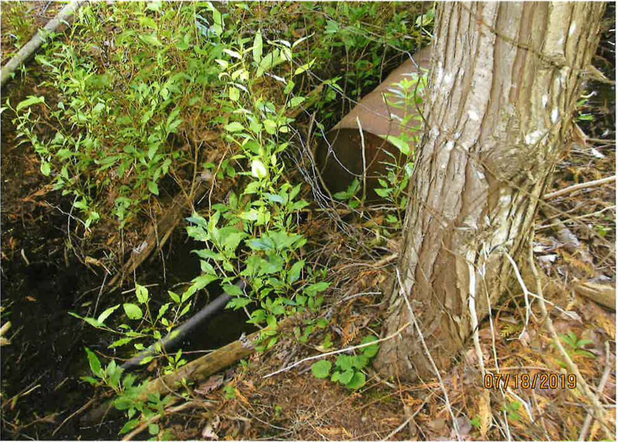
POD – 2 INCH SCREENED POLY PIPE IN BARREL
