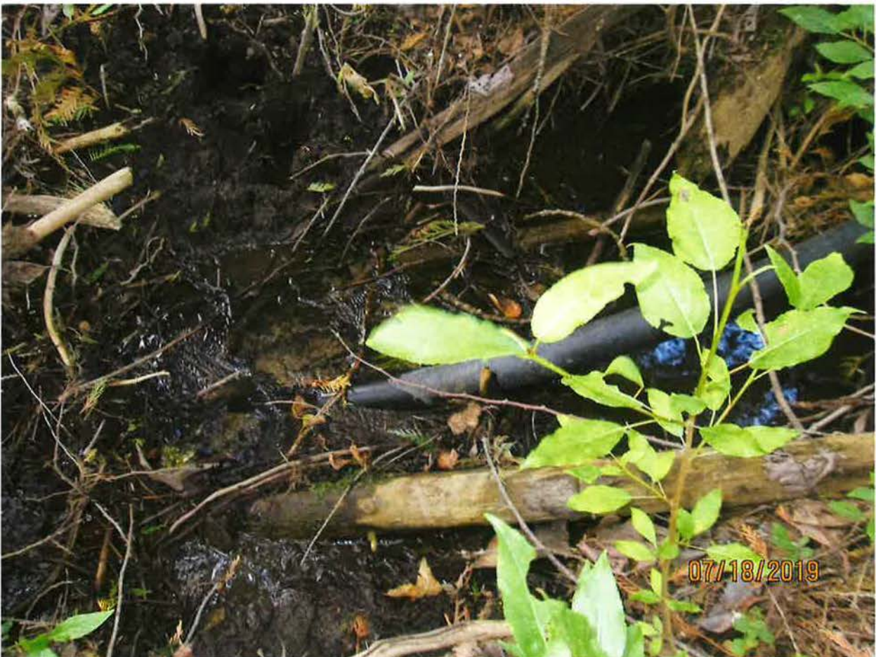
2 INCH POLY PIPE ROUTED THROUGH FOREST FROM POD TO POU
