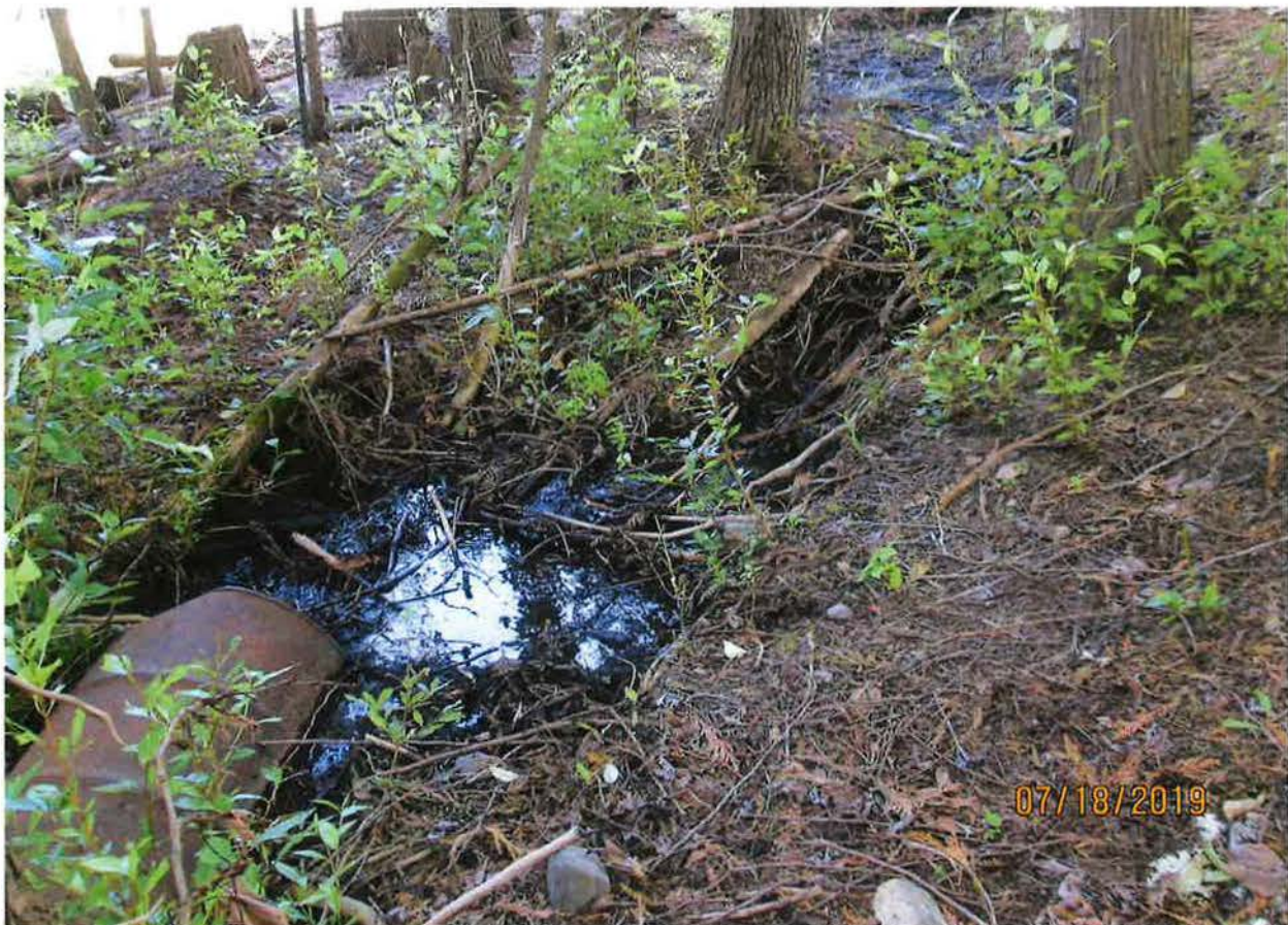
POD – 55 GAL CATCH BASIN IN UNNAMED STREAM WITH 2" INTAKE POLY PIPE
