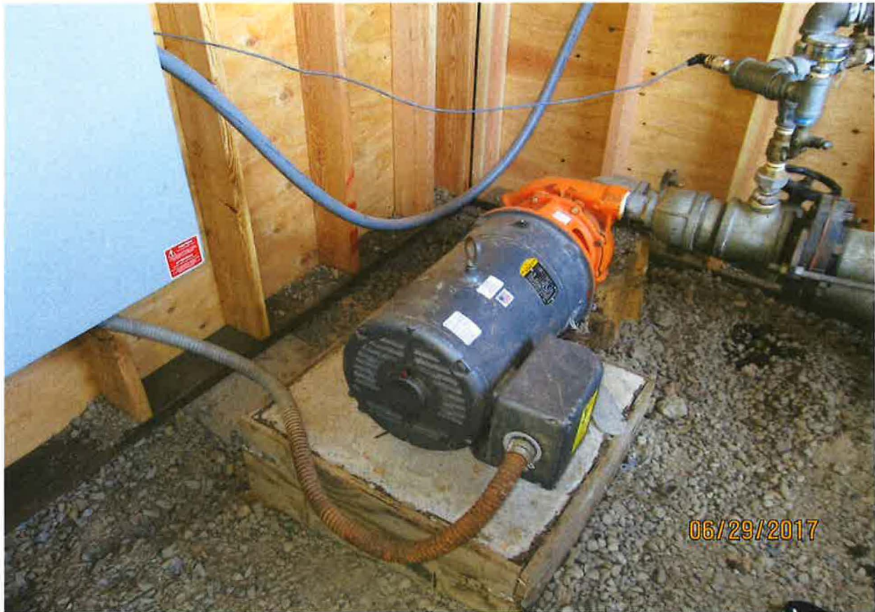
WATER TRANSFER PUMP FOR IRRIGATION FROM STORAGE PURPOSES
