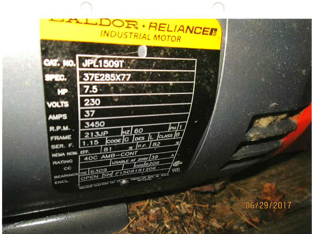
7.5 HP PUMP DIVERTING WATER FROM CREEK TO POND
