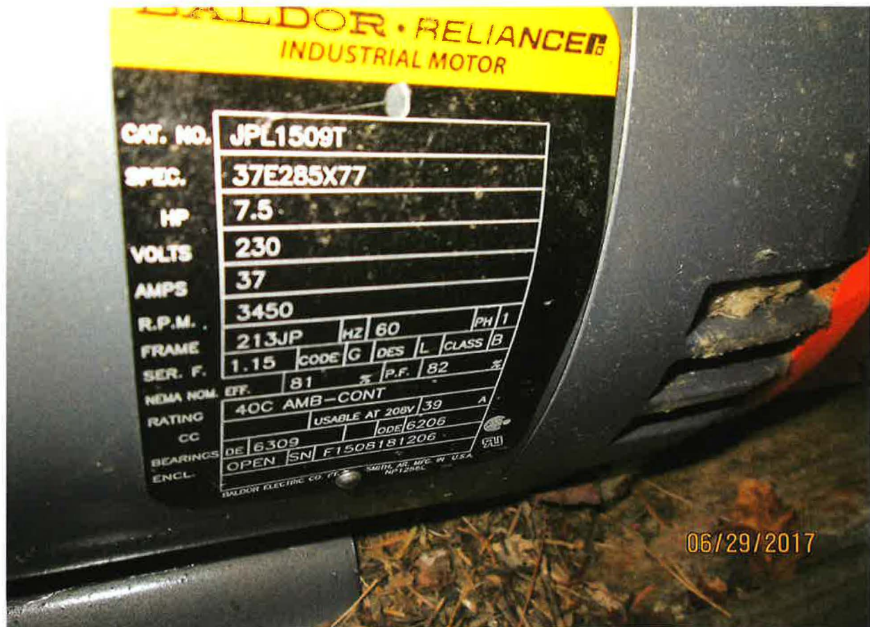
7.5 HP PUMP FOR DISTRIBUTION FROM RESERVOIR TO MUNICIPAL POU
