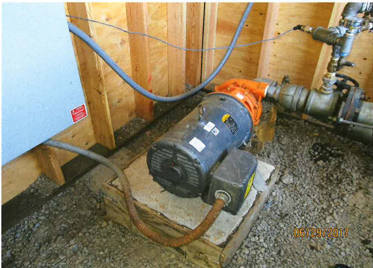
DISTRIBUTION PUMP FROM RESERVOIR
