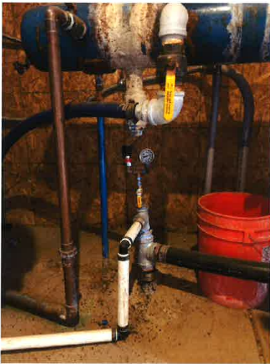
Photo #12 – Site Visit 10/20/2020 Small well has been separated from the south side of the manifold
