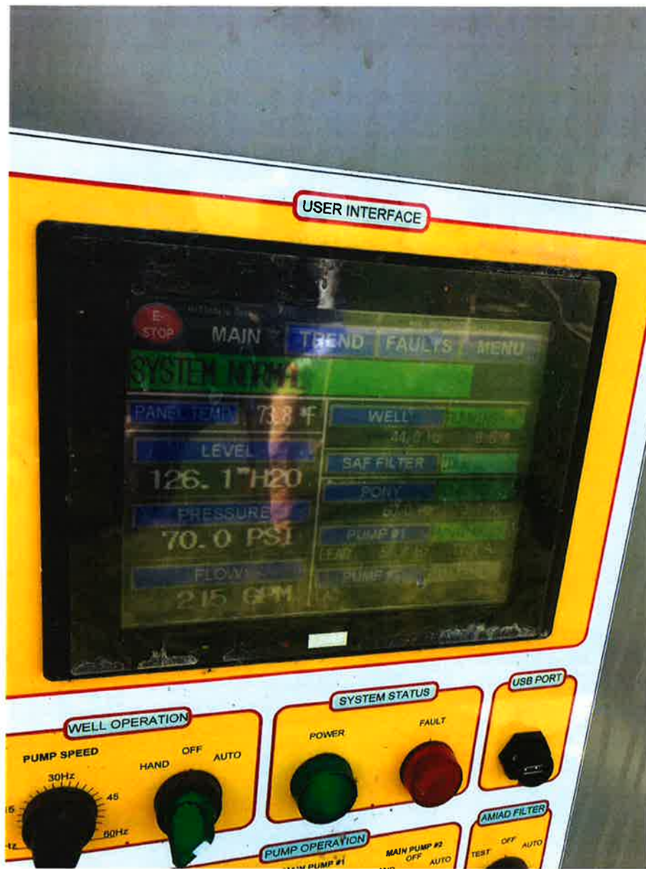
Photo 4. Control panel display showing pumping rate and pressure
