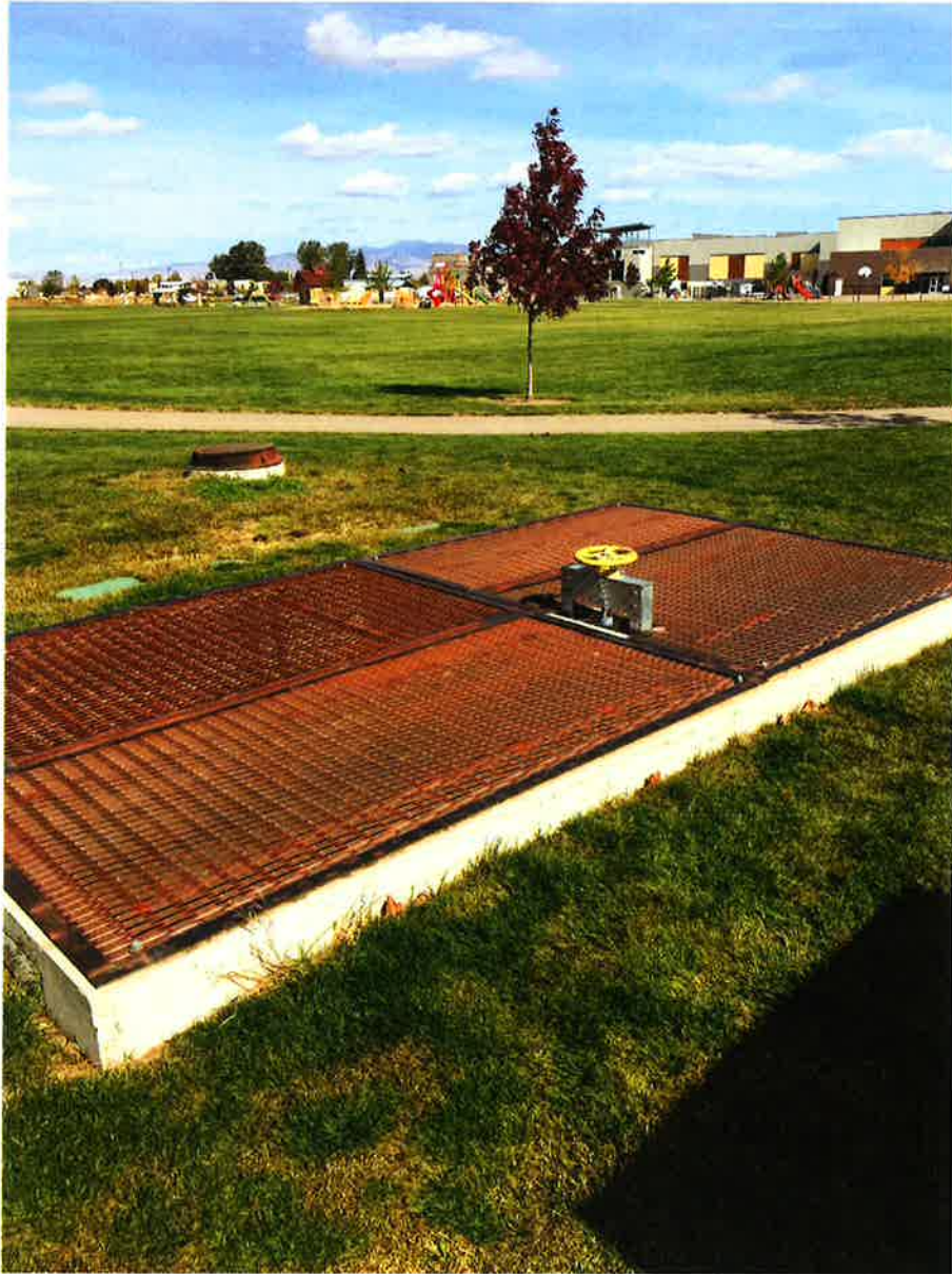
Photo 1. Surface water diversion box, irrigated park in background
