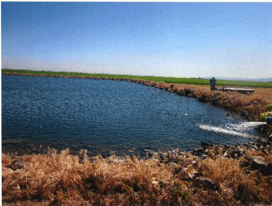
Figure 10: Irrigation pond that is also used for ground water recharge outside of irrigation season (1 of 2 ponds used for recharge)
