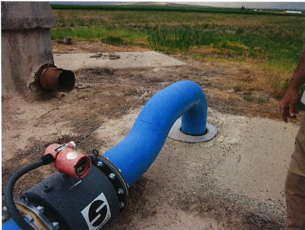
Figure 8: And a third injection well
