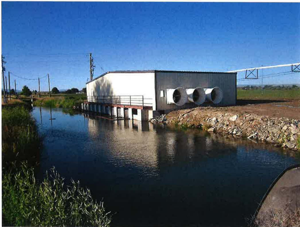
Figure 2: SWID Pump Station
