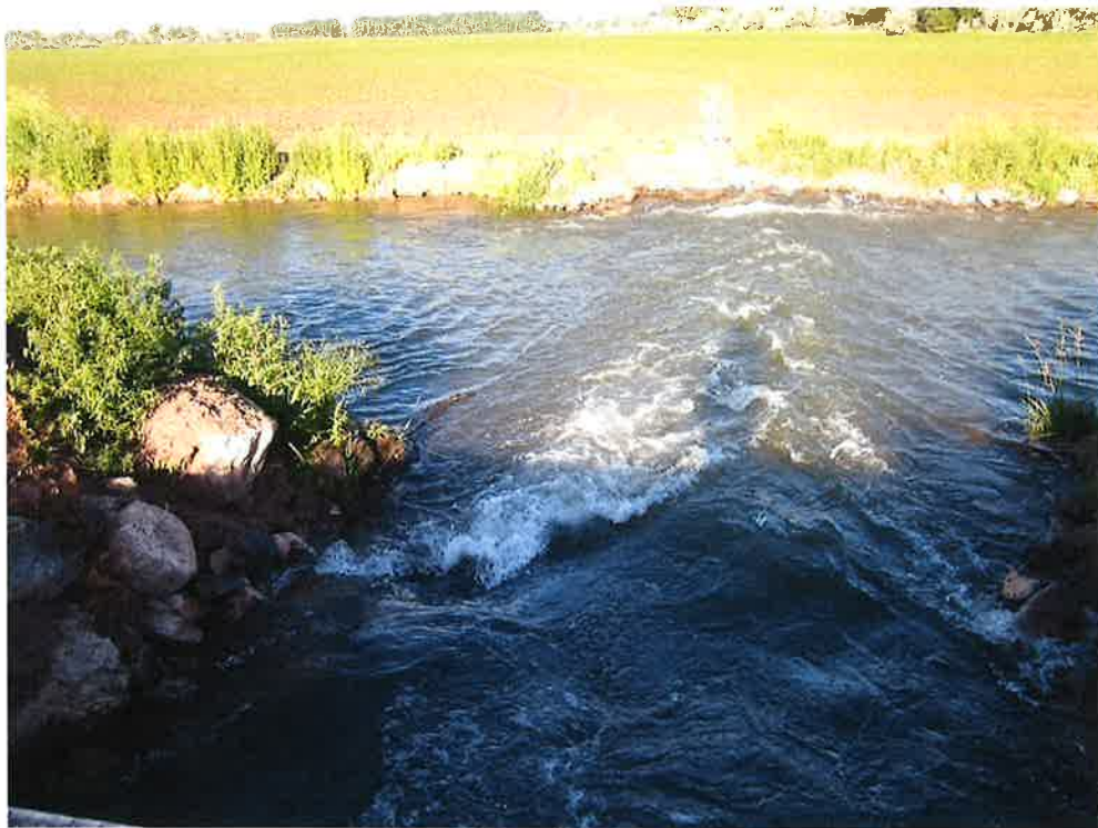
Figure 4: Water diverted from wetland through headgate (Figure 3) into return canal
