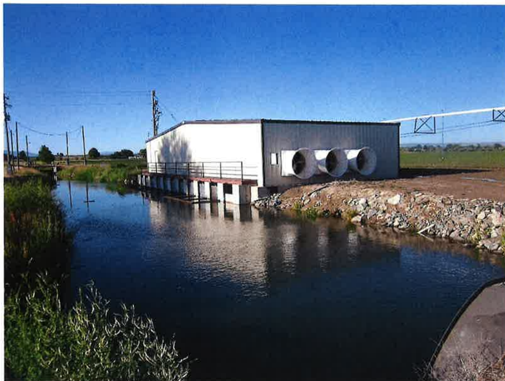
Figure 5: SWID pump station
