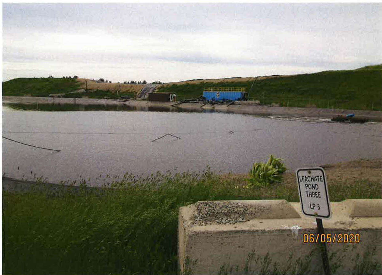
INDUSTRIAL STORAGE POU – LEACHATE POND – LP3
