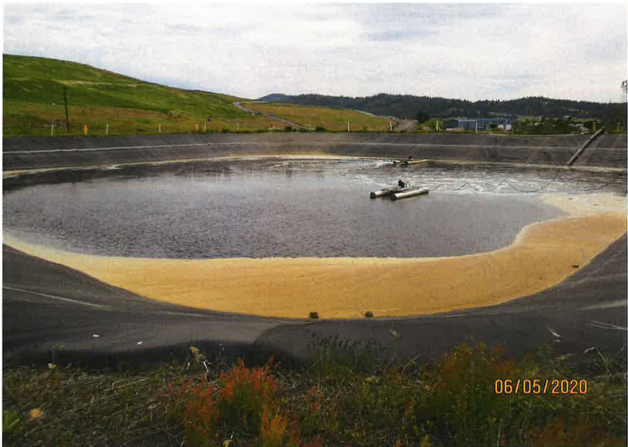
INDUSTRIAL STORAGE, INDUSTRIAL FROM STORAGE, and FIRE PROTECTION STORAGE POU – POND 1B
