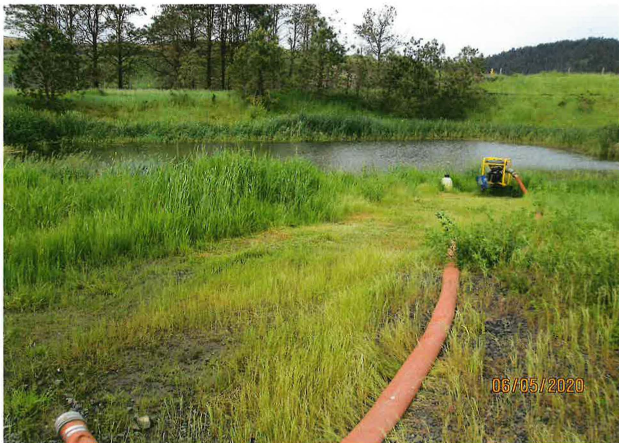
INDUSTRIAL STORAGE, INDUSTRIAL FROM STORAGE, and FIRE PROTECTION STORAGE POU – POND 2A
