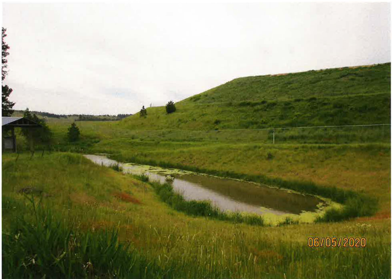
INDUSTRIAL STORAGE, INDUSTRIAL FROM STORAGE, and FIRE PROTECTION STORAGE POU – POND 3A
