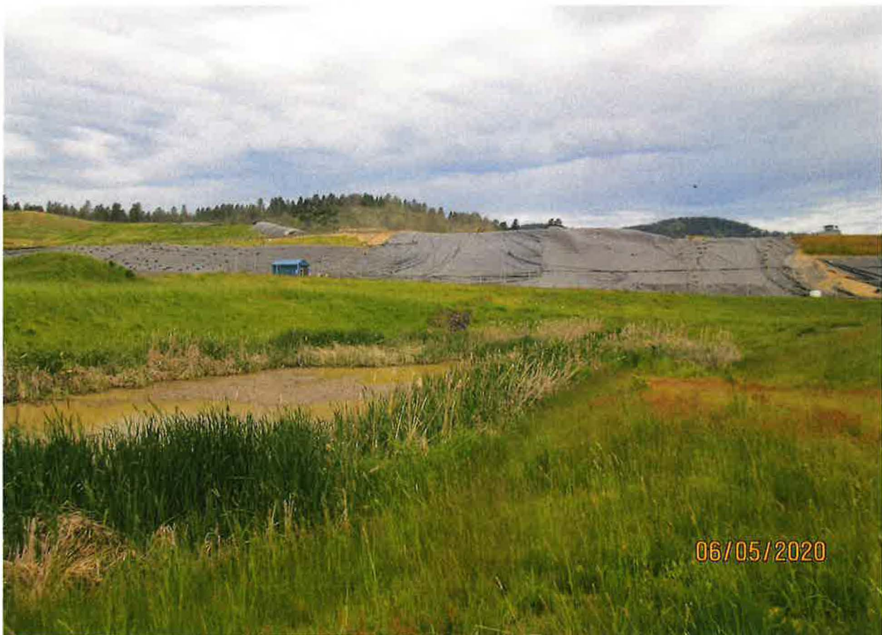
INDUSTRIAL STORAGE, INDUSTRIAL FROM STORAGE, and FIRE PROTECTION STORAGE POU – POND 6A
