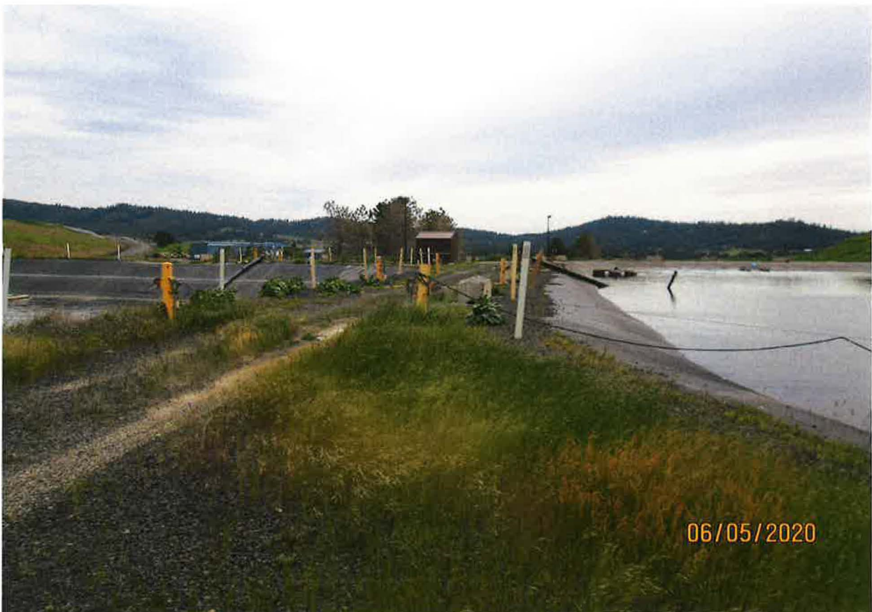
INDUSTRIAL STORAGE POU – LEACHATE POND – LP1 and 2
