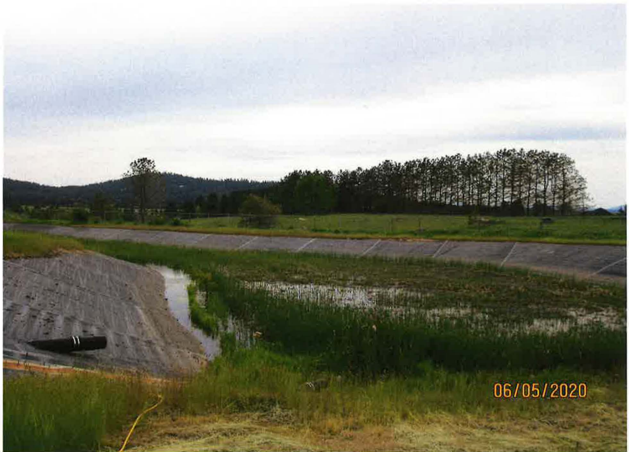
INDUSTRIAL STORAGE, INDUSTRIAL FROM STORAGE, and FIRE PROTECTION STORAGE POU – POND 2B
