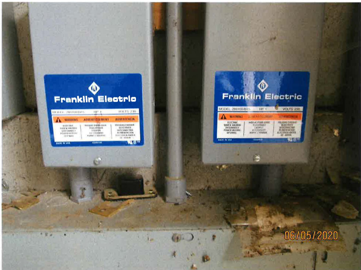
EACH WELL HAS A 1 HP PUMP
