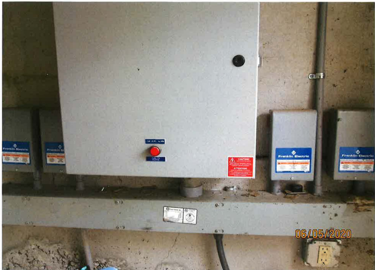
EACH WELL HAS A 1 HP PUMP
