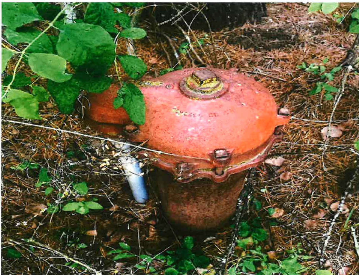
GROUNDWATER POD – WELL 95-87-N-52
