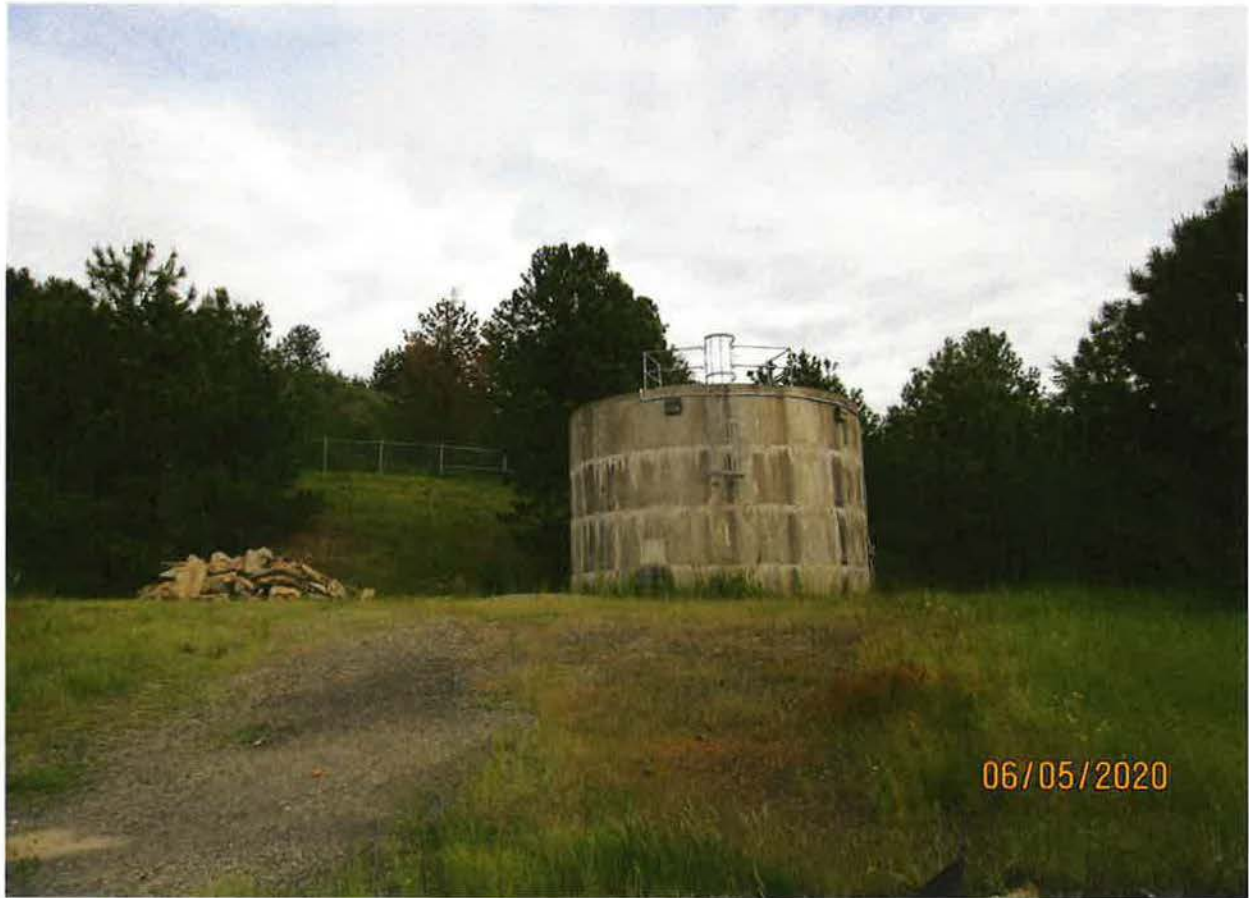
INDUSTRIAL AND FIRE PROTECTION POU – 65,000 GALLON RESERVOIR
